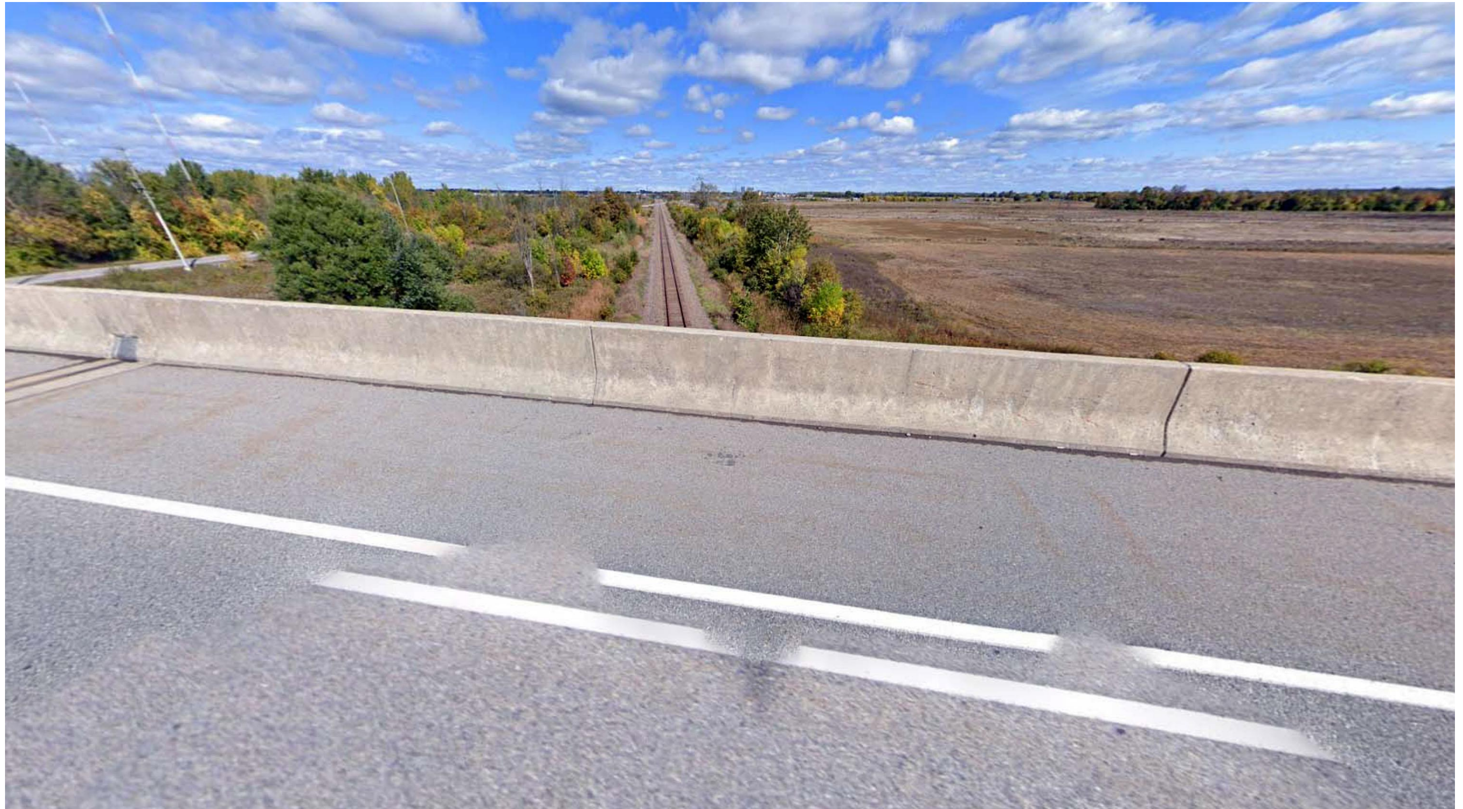
Figure 4: Highway 416 over Railroad Tracks (Photo Source: Google Maps)
