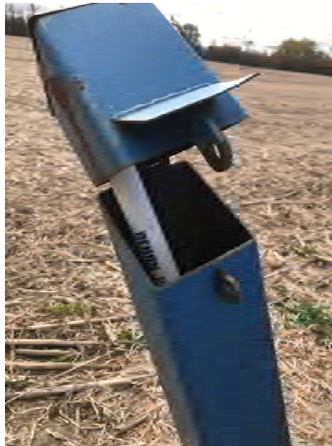
Photo 26 – One of two existing, damaged wells at 4375 McKenna Casey Drive.
