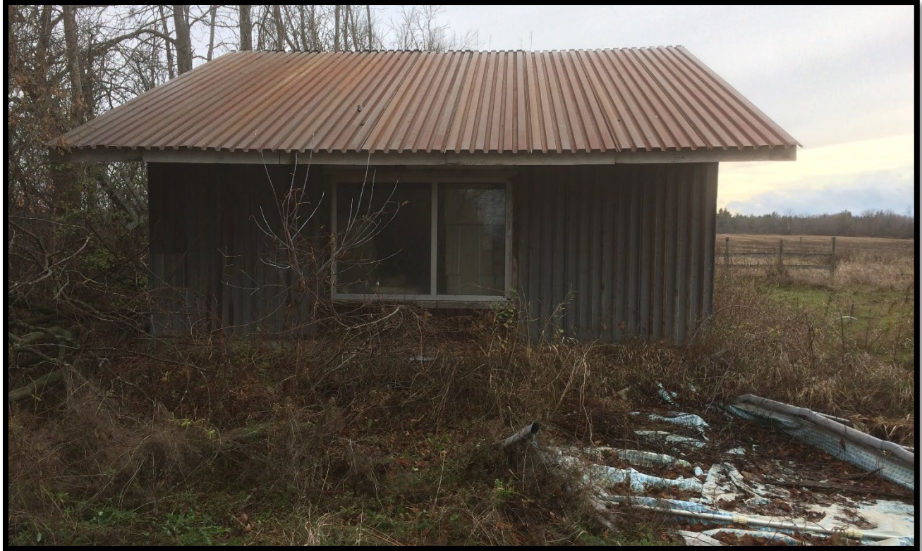
Figure 5: Shed behind residence at 1015 March Road. (PA1156-D34)
