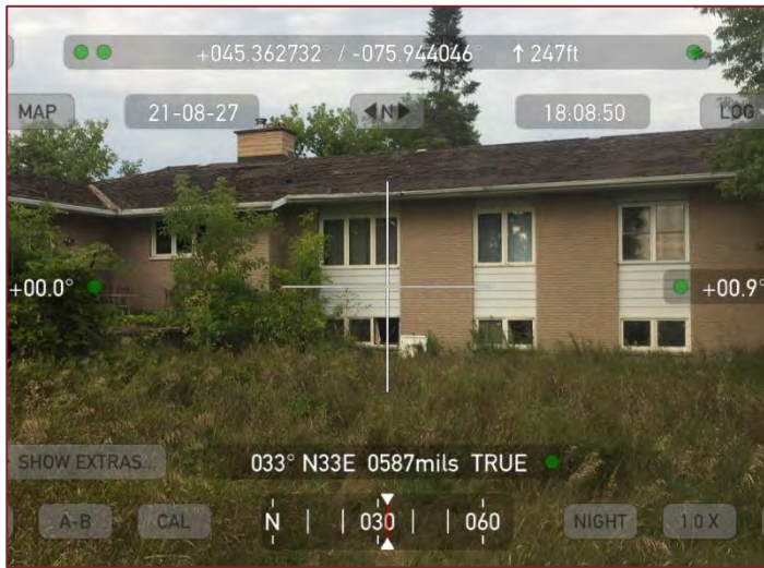
Site Photograph 5 – Existing vacant dwelling
