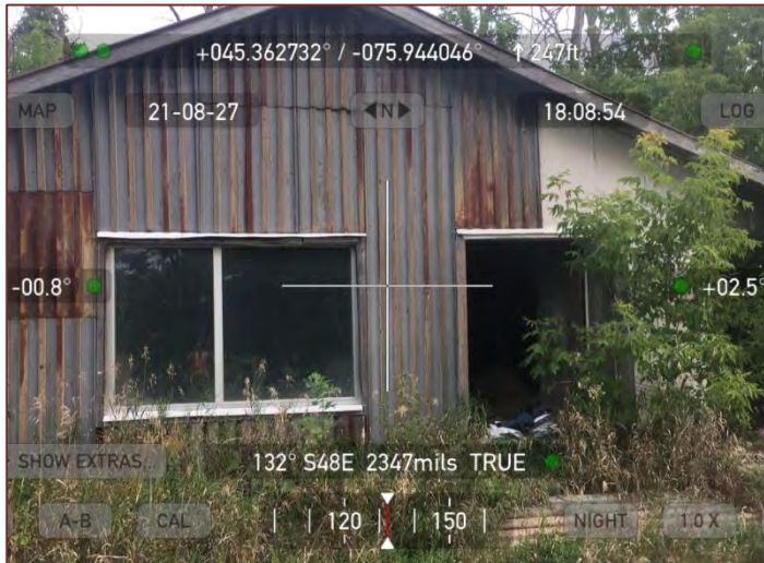
Site Photograph 7 – Existing vacant outbuilding
