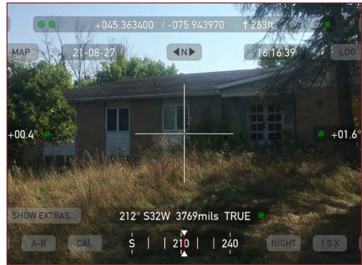
Site Photograph 6 – Existing vacant dwelling
