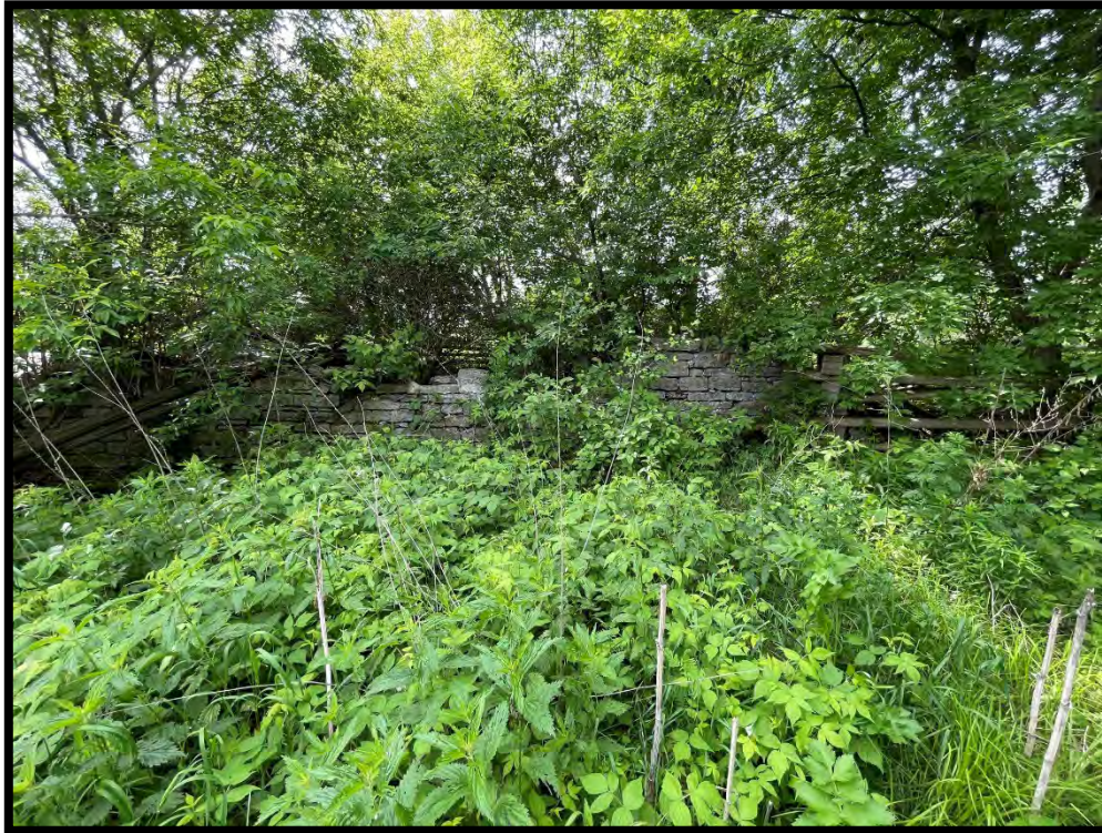
Figure 30: Northern side of collapsed barn (MH1090-D40)
