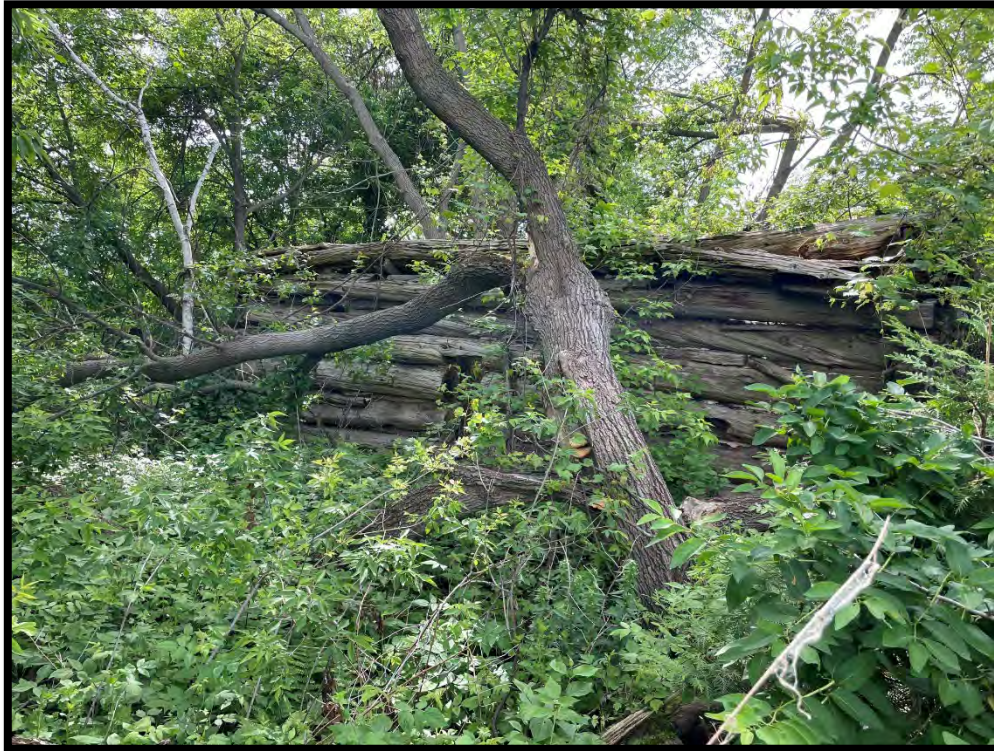
Figure 28: Western side of log structure (MH1090-D30)
