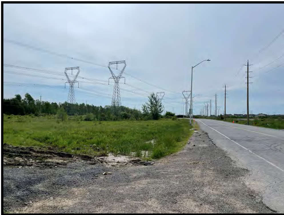
Figure 3: Shea Road along west side with hydro corridor (MH1090-D65)
