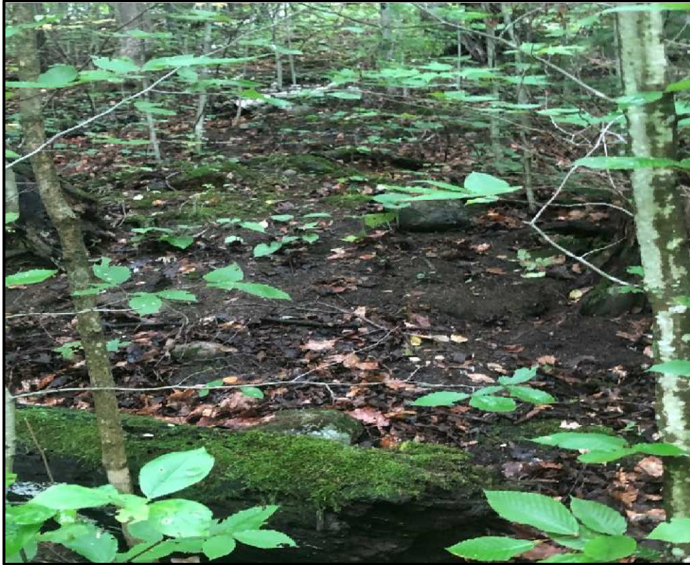
Photo 11A: Photo taken on September 10, 2020 of the south slope face looking southeast near Section O
