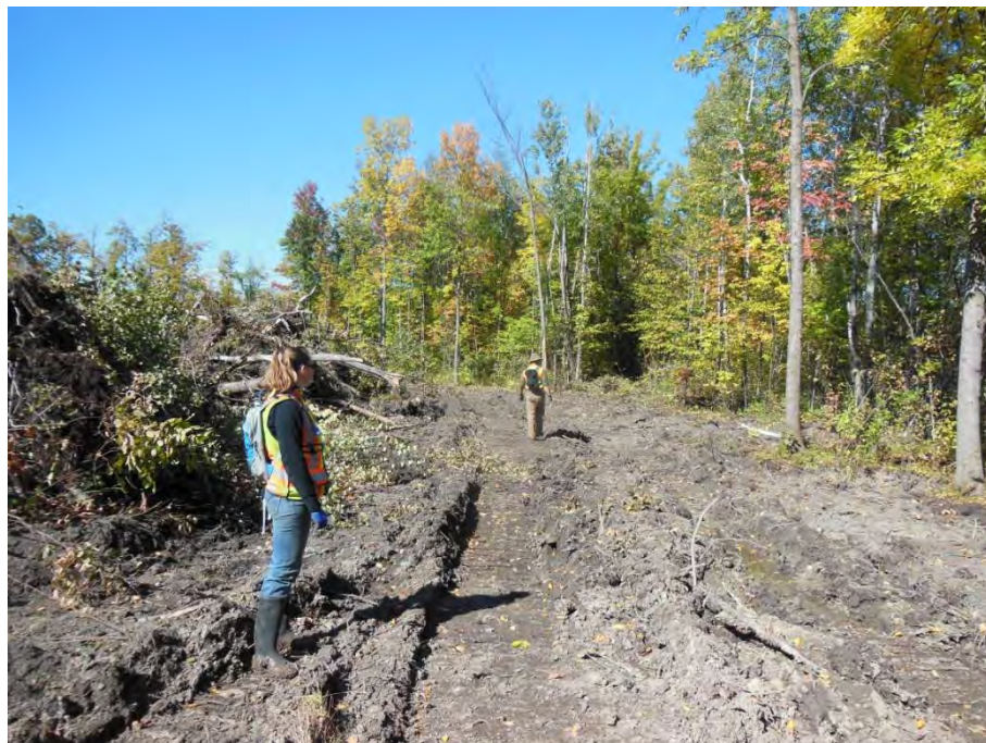
Figure 56: Inspecting grubbed area in Operation 11 (D221).
