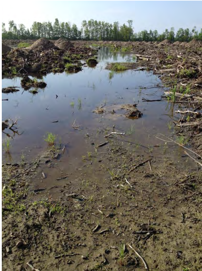
Figure 59: After grubbing on south side (D375).
