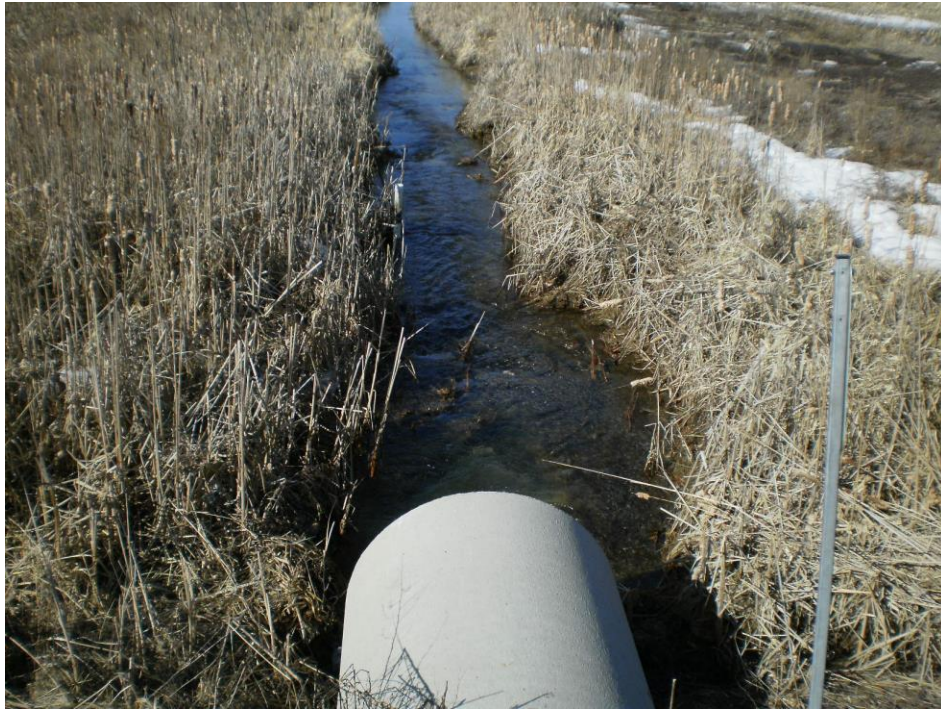
Photo 1 - South tributary looking west from culvert under Cox Country Road (March 17 th , 2020)
