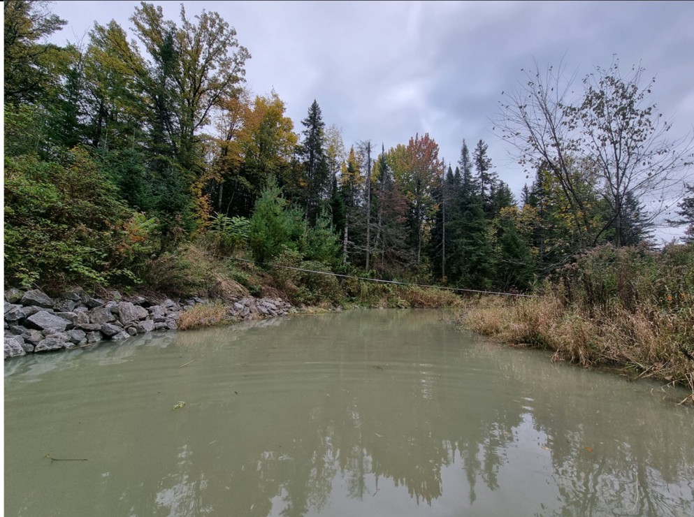
Photograph taken facing upstream at cross-section 5; located upstream of one of three beaver dams observed. Slope stabilization works comprise the right bank around the meander bend for erosion protection.
