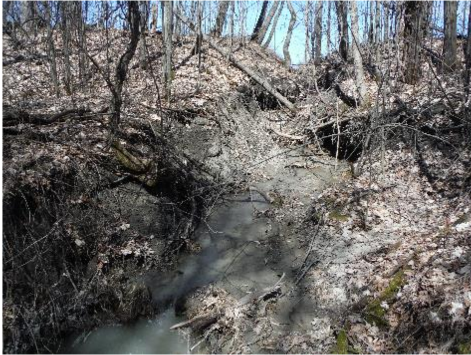
Photo 4: Downstream portion of the North Channel showing the physical barrier (April 6, 2020)
