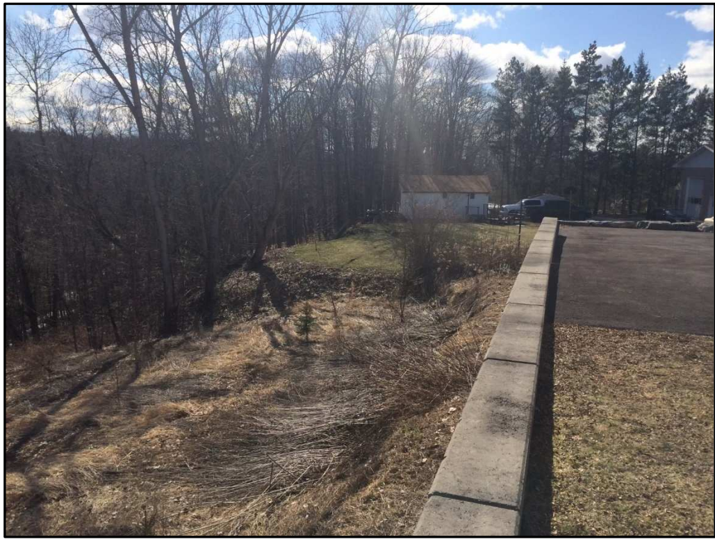
Photo 2: Photograph of failure observed along the top of slope at the property site. Photo taken from the southwest portion of the subject site. Photograph provided by the property owner.
