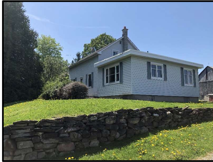
Photograph 1: Front view of the subject property, looking south.
