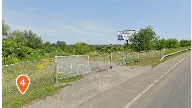
Figure 11: Looking west toward the site at the entrance to the pumphouse
