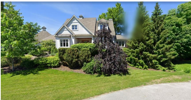
Figure 5: 1101 Antochi Lane, located two lots to the west of the the subject property at 1086 Antochi Lane. This house appears to be set back only 13 m from the river. Source: Google Streetview, image from 2019.
