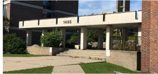
Entrance Canopy and Steps (ERA, 2021)
