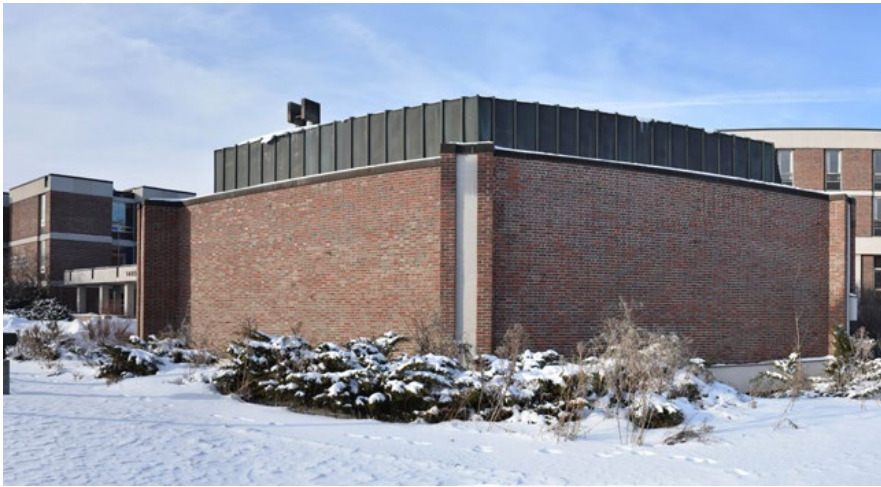
Figure 19. Building F, viewed from southeast (C. Ellis Wong, 2018).
