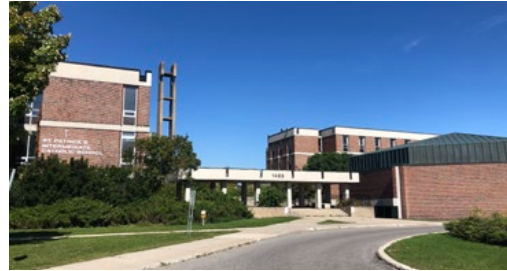
School, Entrance Canopy and Theatre (ERA, 2021)
