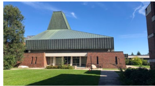
B Courtyard view from the west (ERA, 2021)
