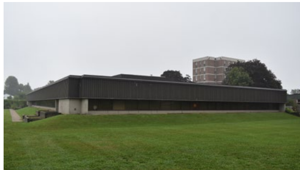
Building M, west elevation
