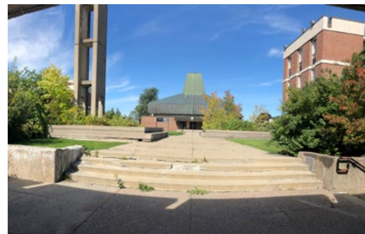
C Terminus view to the Chapel (ERA, 2021)
