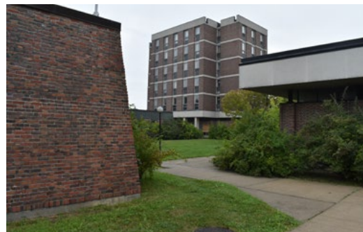
D Academic Courtyard view toward Sisters' Courtyard (ERA, 2021)
