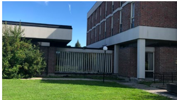
Link between buildings B and C at south elevation
