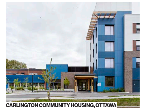
CARLINGTON COMMUNITY HOUSING, OTTAWA Source: GSV Architects
