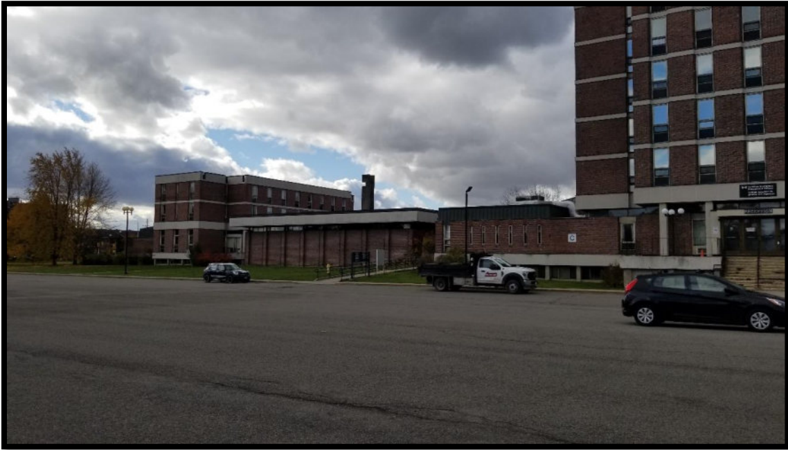
Photograph 1: View of the east facing Site buildings, including Buildings E, D, and C (left to right, facing southwest)
