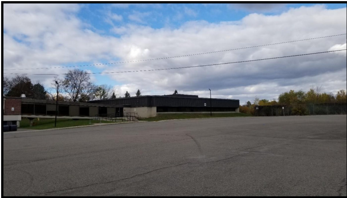
Photograph 6: View of Building M, at the north end of the complex (facing north-west).
