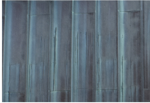
Figure 22. Standing seam copper roofing (ERA, 2021).
