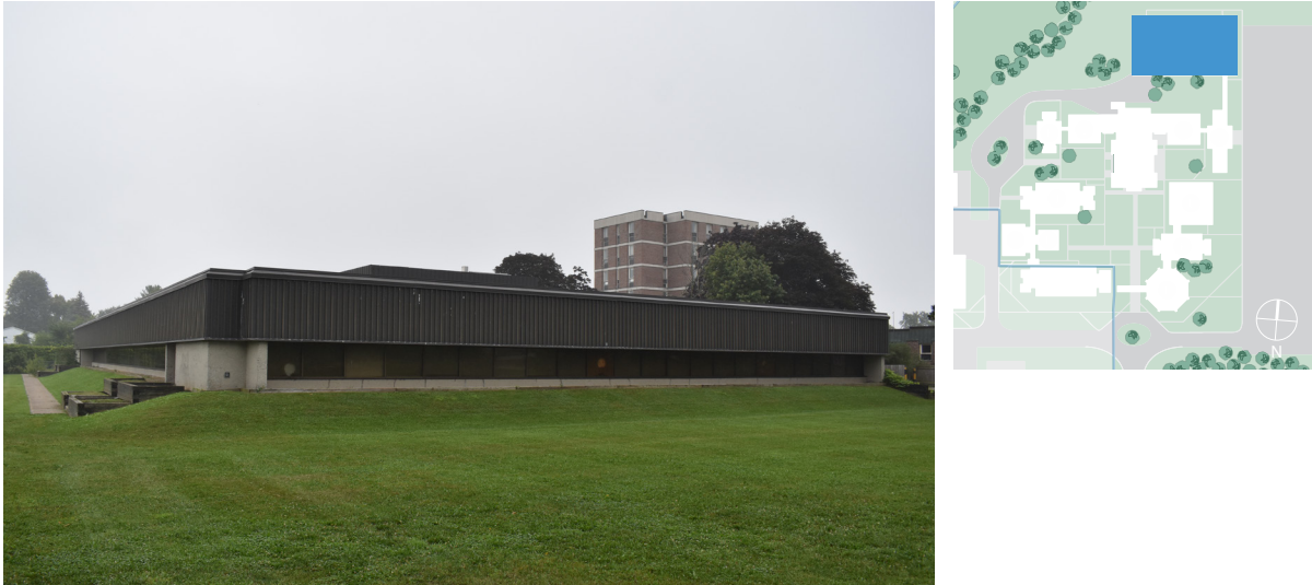
Figure 10. Building M, west elevation (ERA, 2021).
