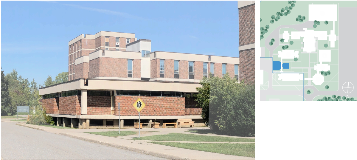
Figure 8. Building I viewed from southwest (ERA, 2021).
