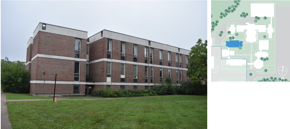
Figure 9. Building J, from Sisters' courtyard (ERA, 2021).
