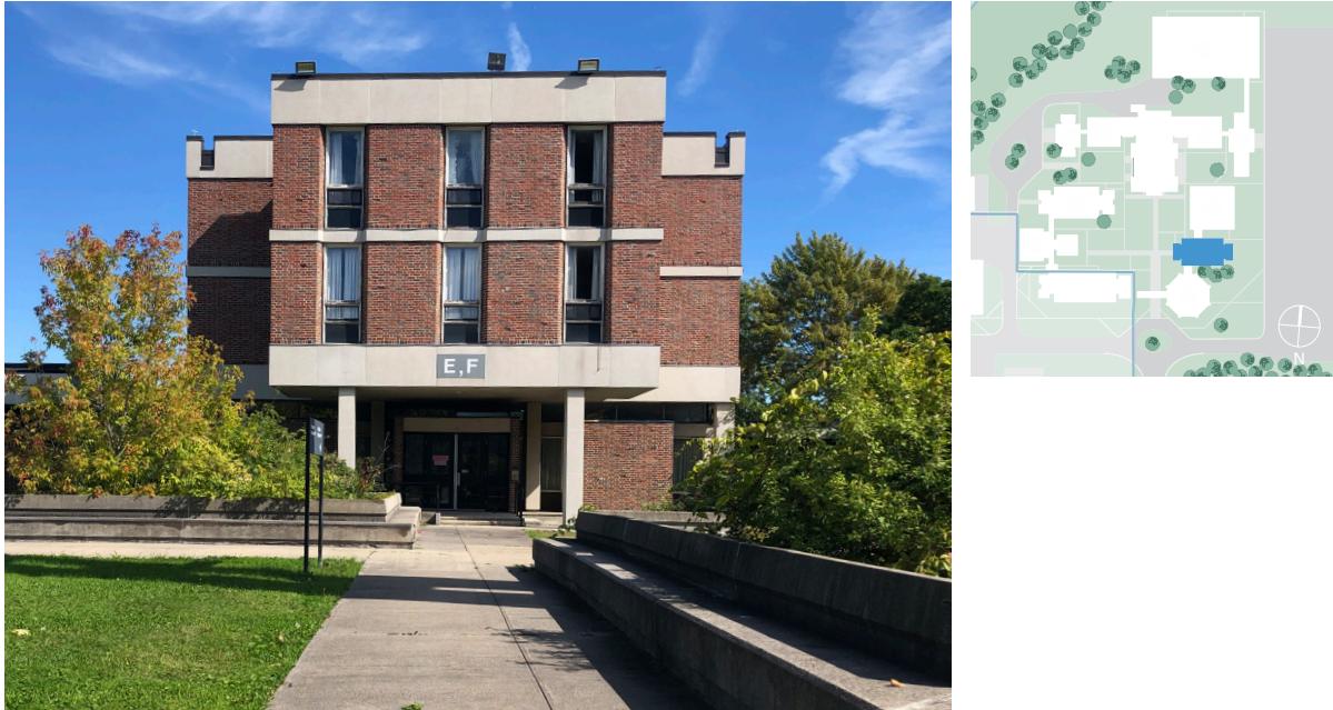
Figure 6. Building E, west elevation (ERA, 2021).
