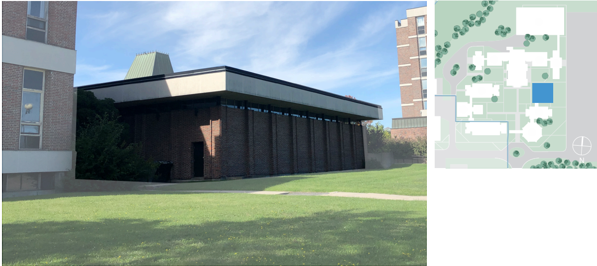
Figure 5. Building D, viewed from southeast (ERA, 2021).
