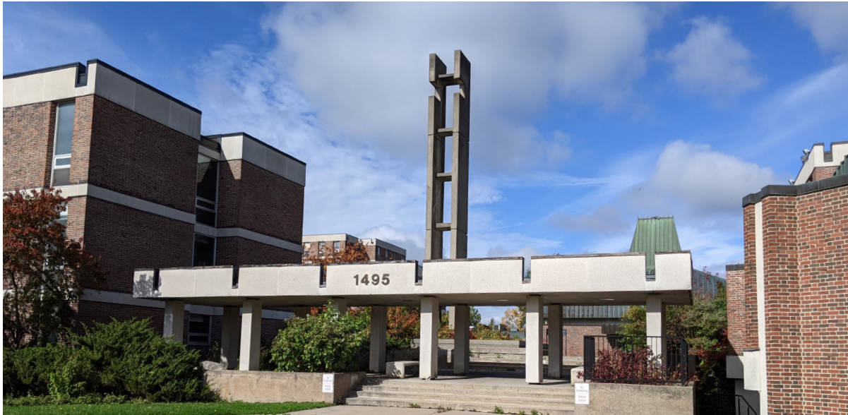
Figure 12. Main entrance canopy, with Campanile behind (ERA, 2021).
