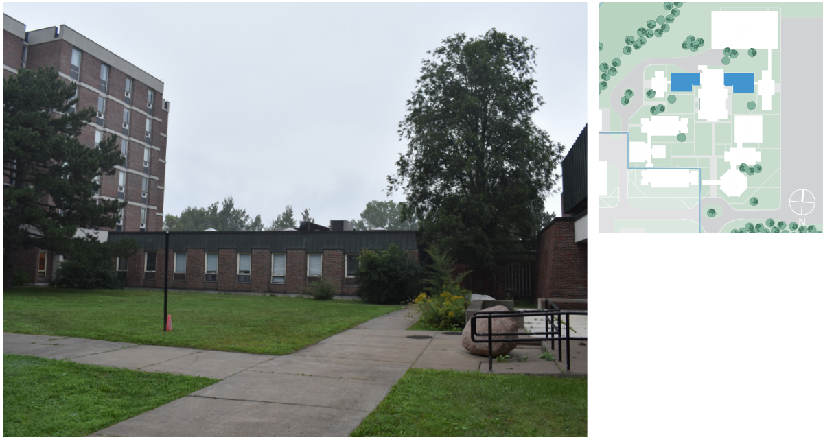
Figure 3. Building B, from Sisters' courtyard (ERA, 2021).
