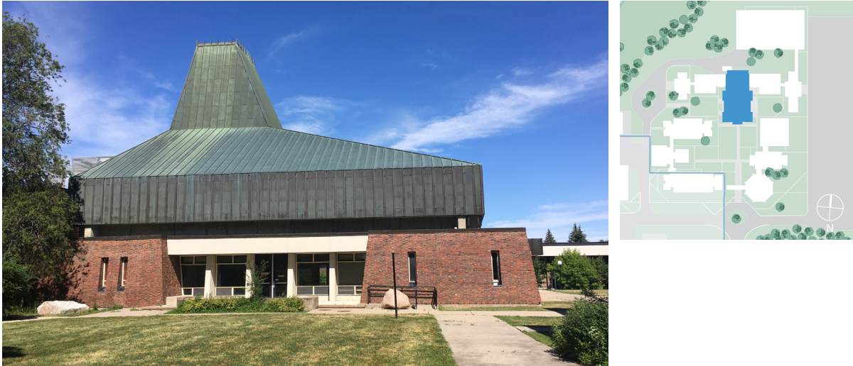
Figure 2. Building A, west elevation (ERA, 2021).
