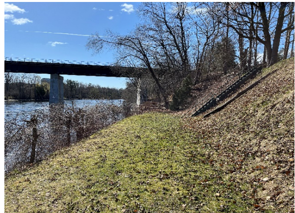
View 4 looking south at eastern edge of the site showing embankment to the river and elevated track.
