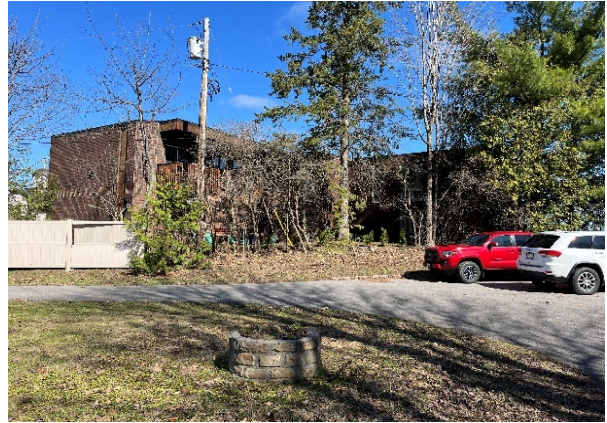
View 2 looking north on northeastern edge of site.
