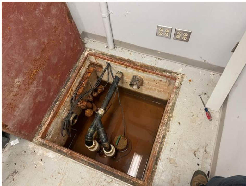
Photo 8: Sump pit in storage room in 603 March Road.
