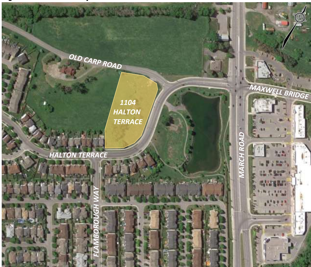
Figure 1: View of the Subject Site
