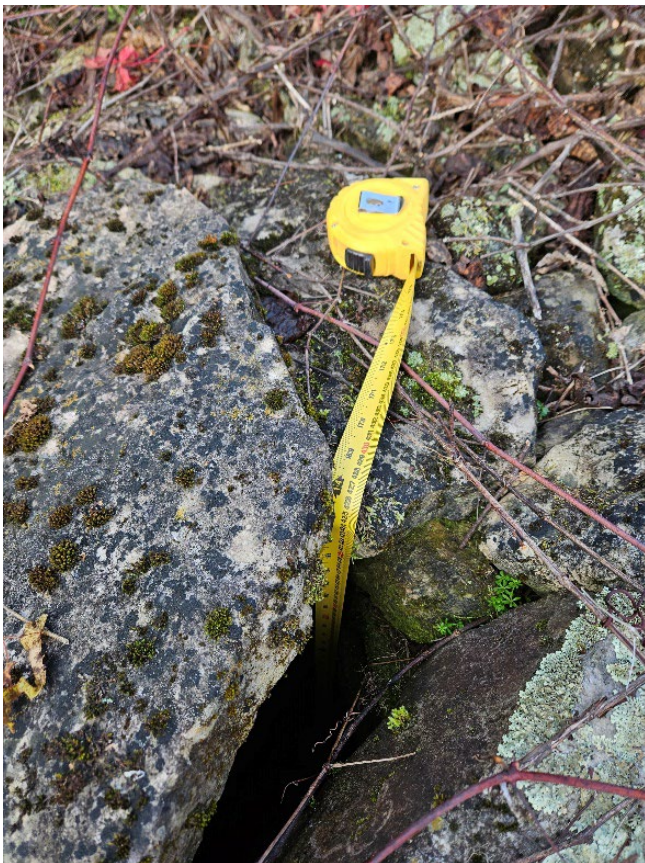
Image 10: Void measuring 4.25 m below the surface within the well, looking west.
