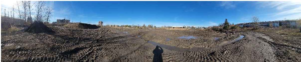
Figure 8 Site condition after earth moving occurred as part of remediation efforts
