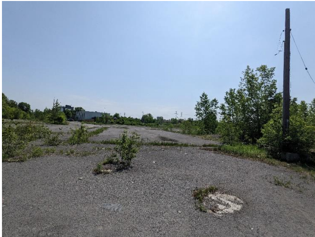
Figure 7 Site condition prior to significant earth moving occurred on the lands
