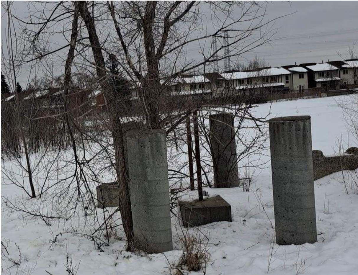
Photograph No. 5: Existing Tree with Concrete Posts
