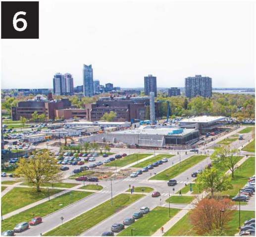
View of new ESAP building
