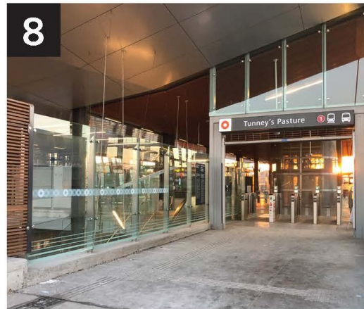
Tunney's Pasture LRT Station entrance
