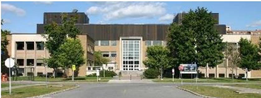
Figure 4 - Statistics Canada Building
