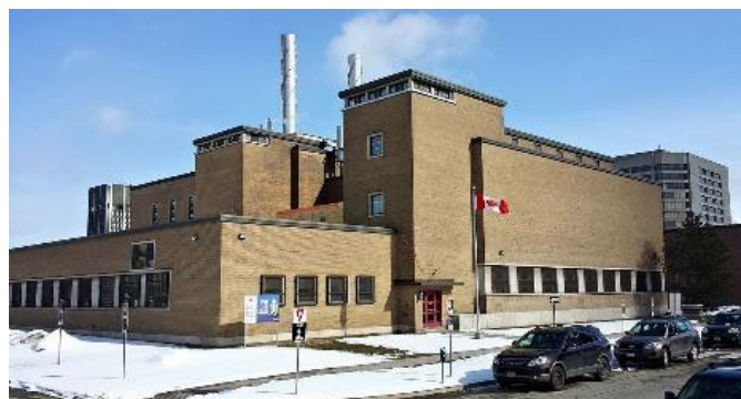
Figure 7 - Central Heating and Cooling Plant
