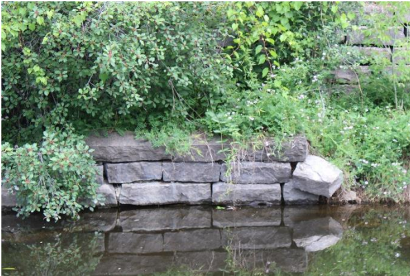
Photo 4.19: Damage to stone wall
