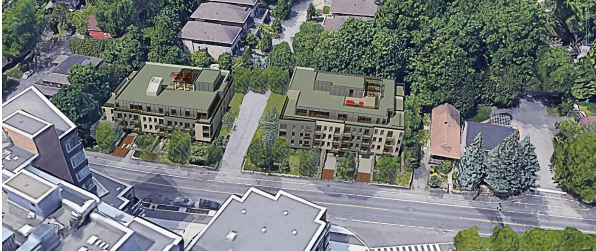
Figure 30: Using variations in the setbacks, the façades are broken down to suggest the original lots and to maintain the residential character of the site. Because the basement is partially exposed along Beechwood the height is consistent with others along the street whereas the 3 and 4 storey height along the rear relates to the residential units along Carsdale. As with a number of Rockcliffe homes, taking advantage of grade changes to allow for walkouts is a common practice.
