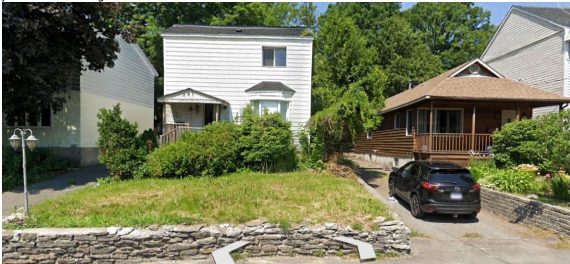
Figure 16: Street view of the circa 1950 two-storey single detached properties at 245 (left), and 247 (centre) Beechwood Avenue built to standard plans developed by the CMHC. The small cottage-style residence at 249 (right) Beechwood is not part of the proposed development. Note the stone retaining wall at the street, and the simple landscape treatment. Source: Google Earth
