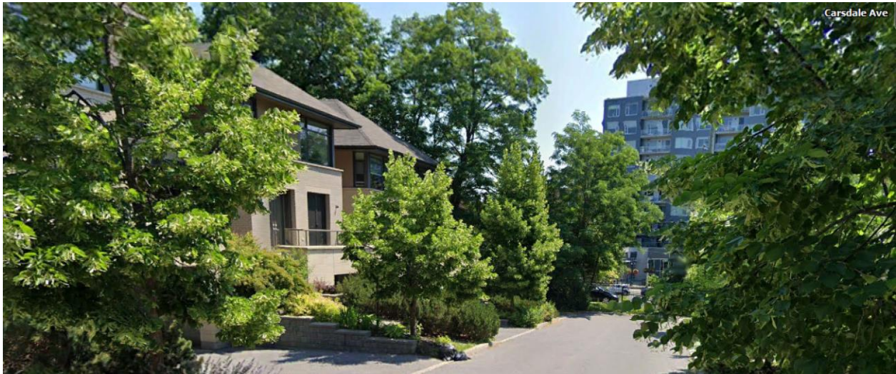
Figure 7: Street view looking east on Black Maple Private/Carsdale to the west of the development site. Source: Google Earth
