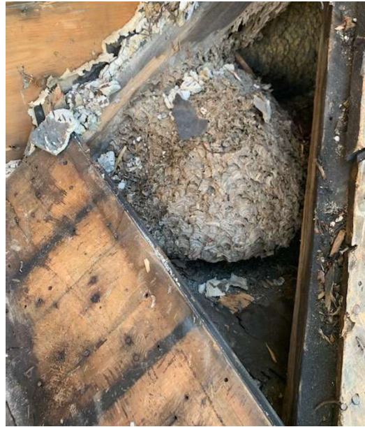
Fig. 12 and Fig. 13: As flashing was not used in original construction, crown mouldings and boards were subject to rot over the years leaving gaps where squirrels, birds and wasps were able to enter and nest
