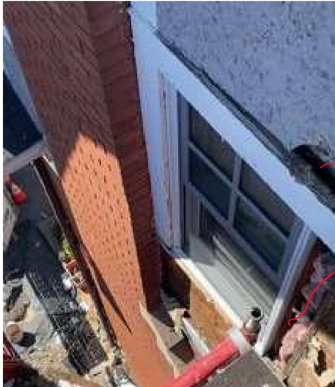
Fig. 14: Inadequate insulation at all windows
