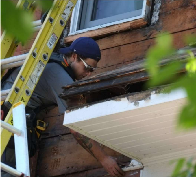
Fig. 12 and Fig. 13: As flashing was not used in original construction, crown mouldings and boards were subject to rot over the years leaving gaps where squirrels, birds and wasps were able to enter and nest
