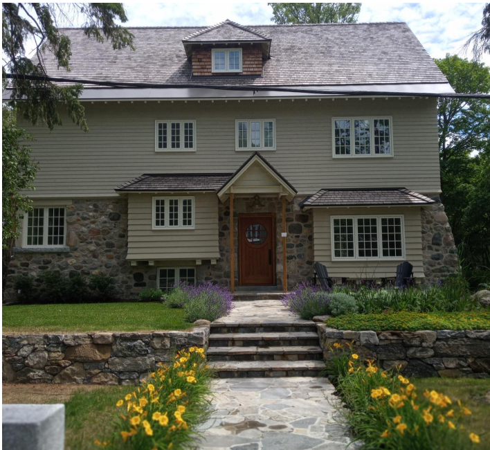
Figure 33: View of the front entrance walk with the new dry stone retaining wall and raised terrace. The wall is a beautifully executed example of masonry work. Source: Commonwealth 2021.
