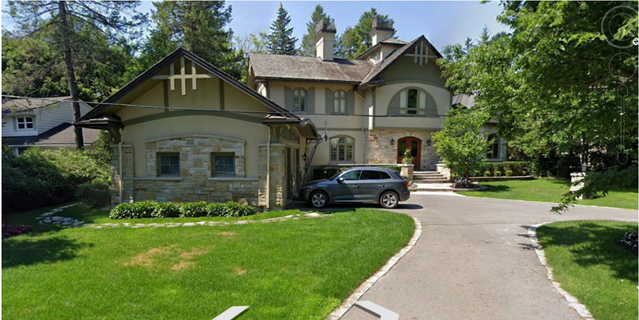
Figure 10: Street view of 16 Crescent Road next to 14 Crescent Road whose roof is visible to the left of the image. The property is an example of recent infill development. The placement of the garage in the front yard of the property and the semi-circular driveway are common features of properties along the crescent. Source: Google Earth 2019.
