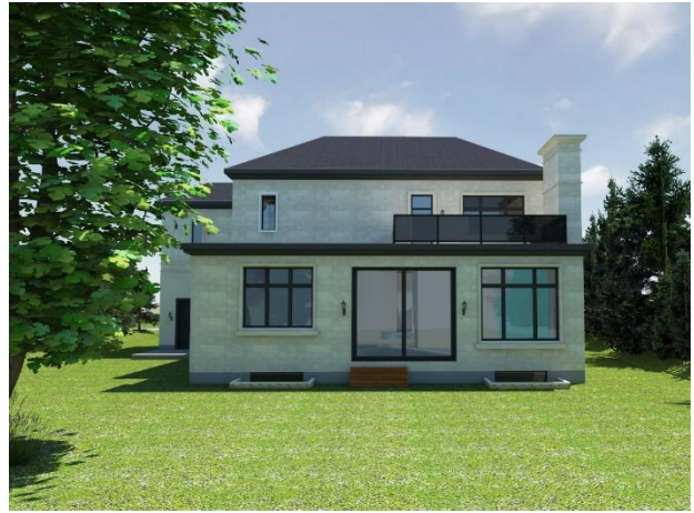
Figure 8: West elevation – rear façade
