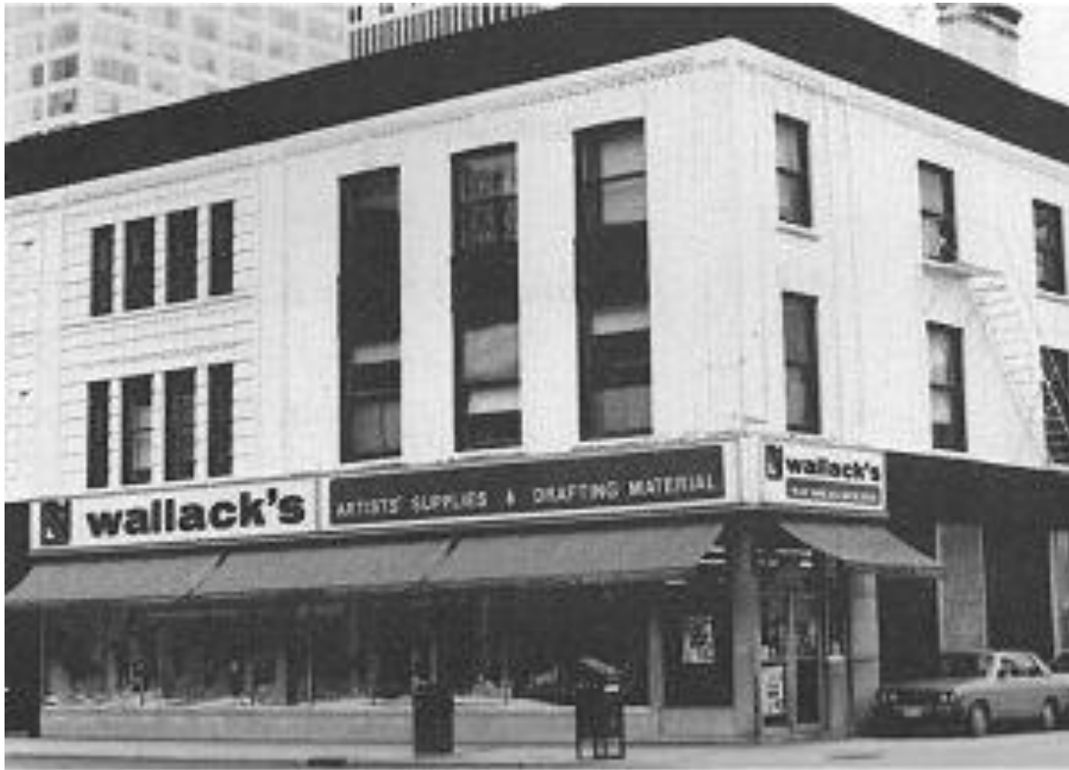
Figure 19: A view of 231 with the retail entrance shifted from its original central location to the corner and the upper façade painted white. A black band can be seen between the ground floor retail and the upper floors.
