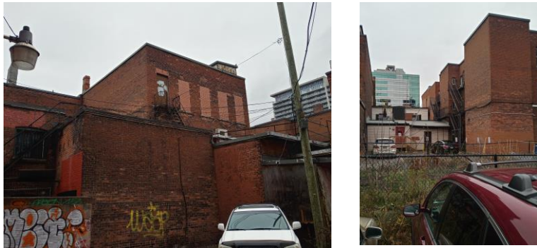
Figure 16: Views of the east façades (rear).
