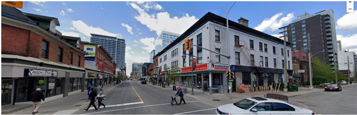
Figure 8: A street view looking north-east, with the Wallack Building holding the Lisgar Street corner on the east and a 2.5 storey retail unit across the street. Next to it is the 1-storey Comic Shop.
