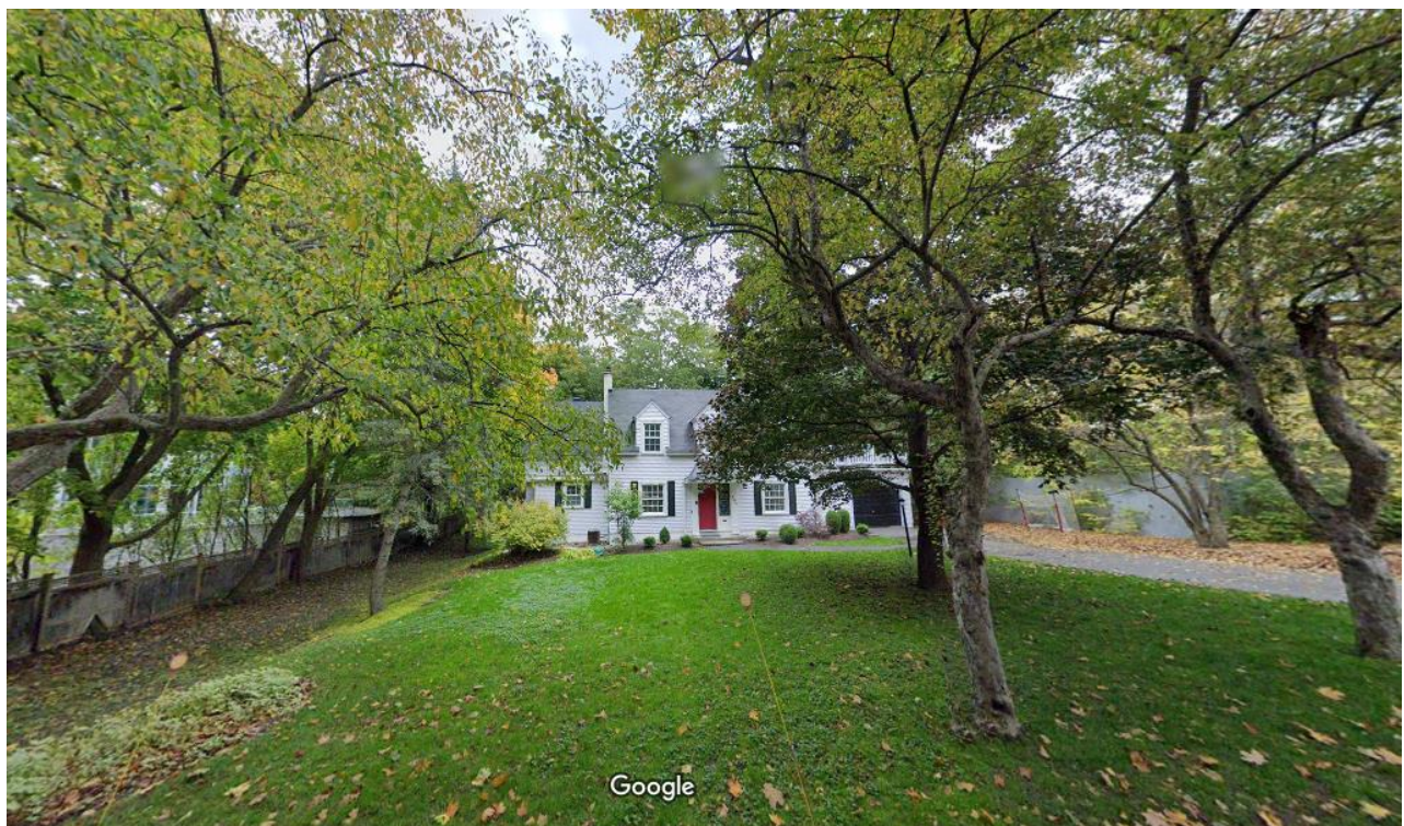
Figure 6: View of 484 Cloverdale Road to the north of the development site. The property is a 1 1/2 Storey Grade 1 contributing property within the context of the HCD. The front yard with fruit trees and manicured lawn are defining features of this property and support the picturesque traditions of the HCD as seen from the street. A two-storey addition in the rear yard takes up most of the soft landscape and presents a much larger footprint than is suggested from the street. Source: Google Earth.
