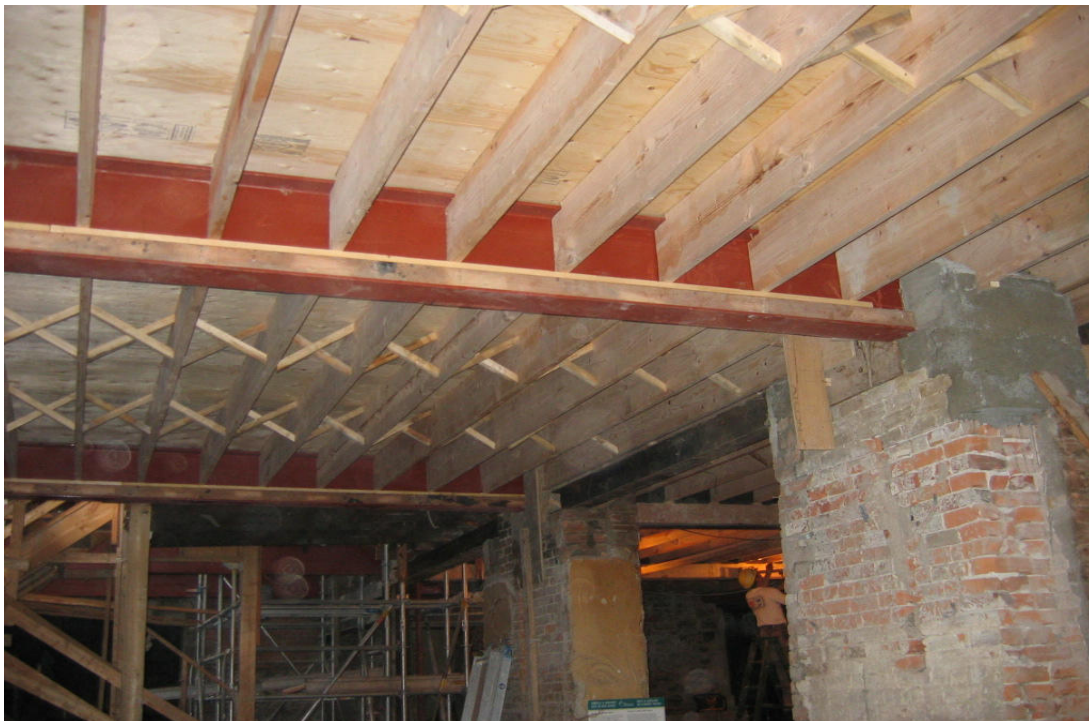
Figure 7: Previously Existing Condition Outlining Brick Piers in Basement
