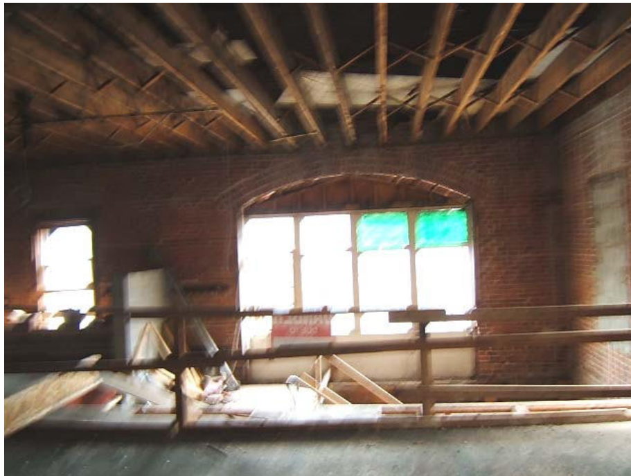
Figure 9: Previously Existing Condition Outlining Roof Diaphragm
