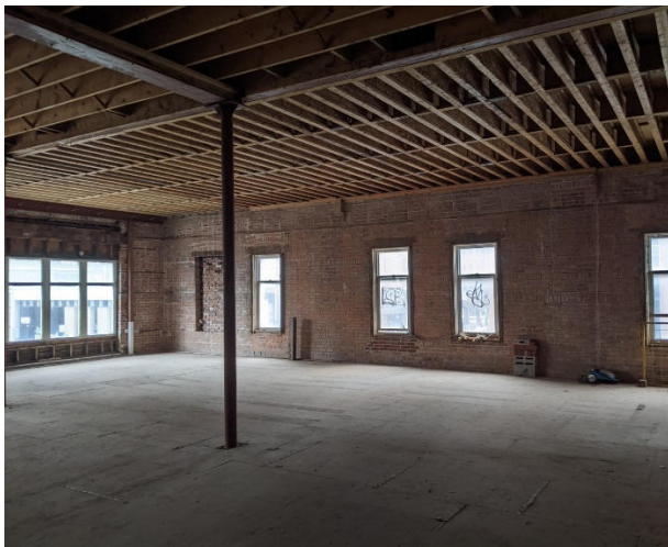
Figure A7 – Second Floor Facing North
