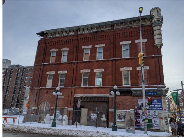
Figure A2 – North Exterior Wall
