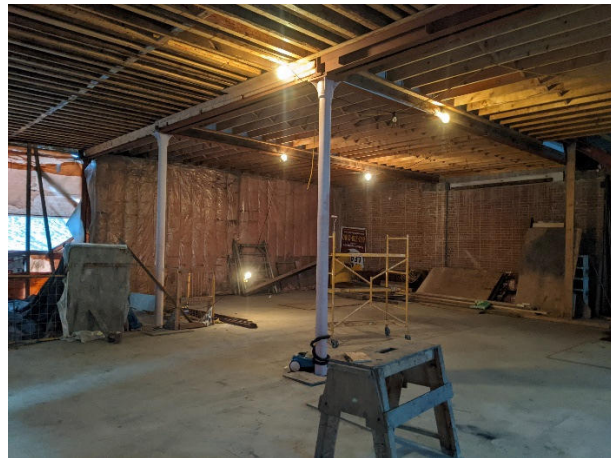
Figure A4 – Ground Floor Facing East
