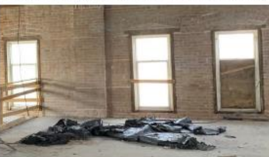
Figure 34: Interior of third floor windows on the north façade.
