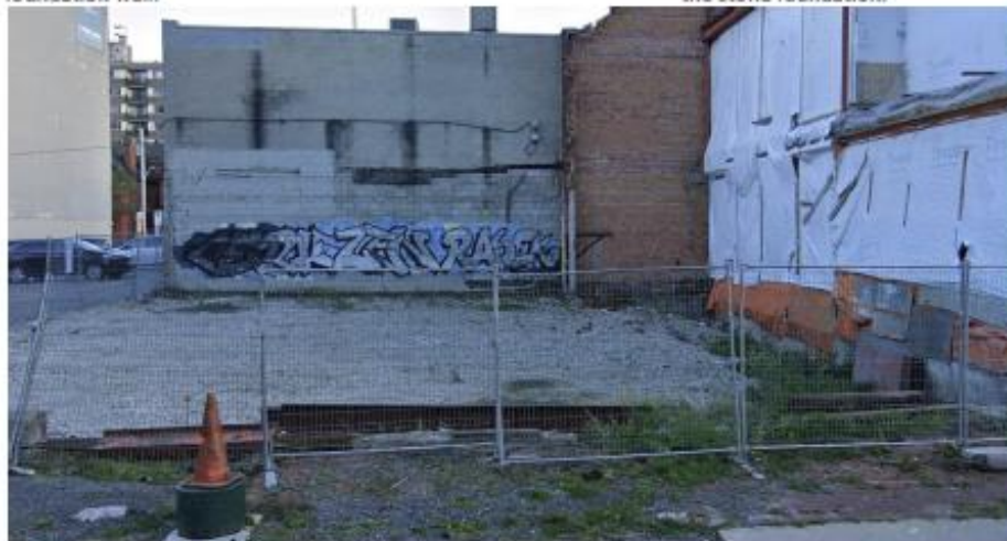
Figure 53: Backfilled location of previous addition, sloping towards the remainder of Somerset House.
