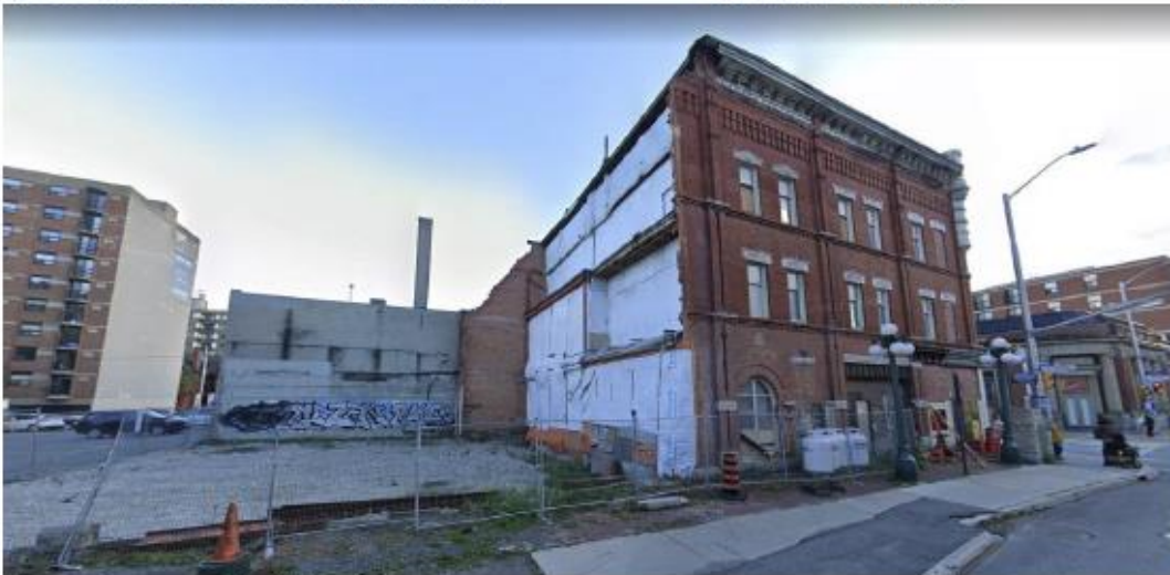
Figure 5: Current state of the building
