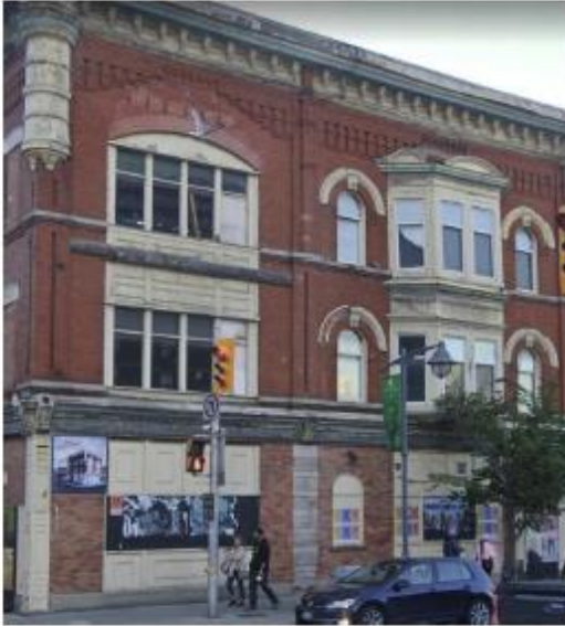
Figure 21: Openings on the west façade.
