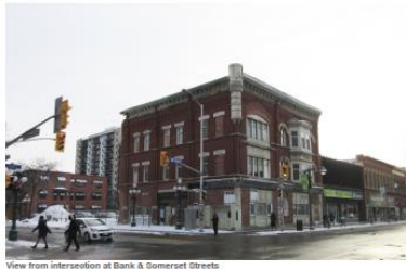
View from intersection of Bank & Somerset Streets
