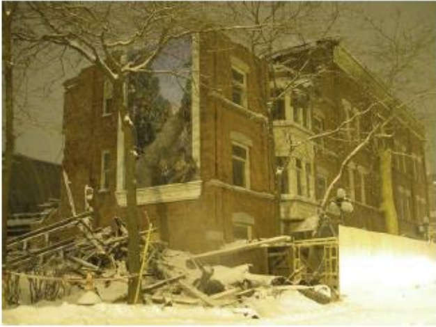
Figure 3: Somerset House after 2007 partial demolition
