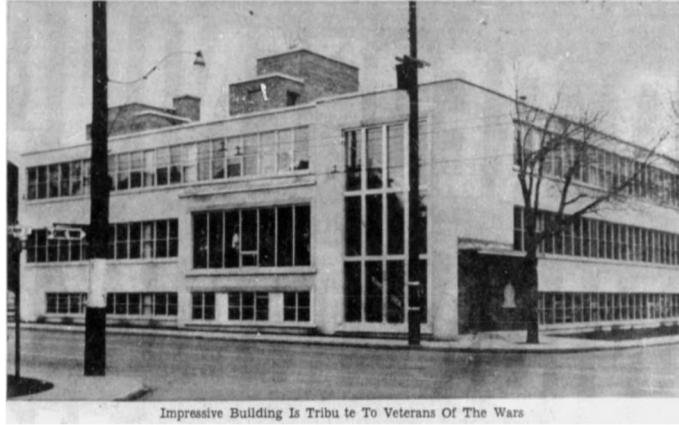
Figures 2 The Legion House as it appeared in 1955 . The limestone veneer and the horizontal banded fenestration with aluminum trim are features that were carried into the 1958 addition. These prominent attributes will to be conserved.
