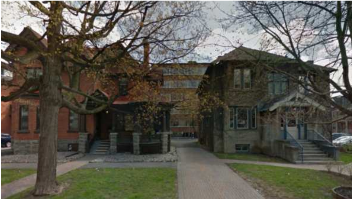
Figure 31: View of 436 (left) and 444 (right) MacLaren Street.
