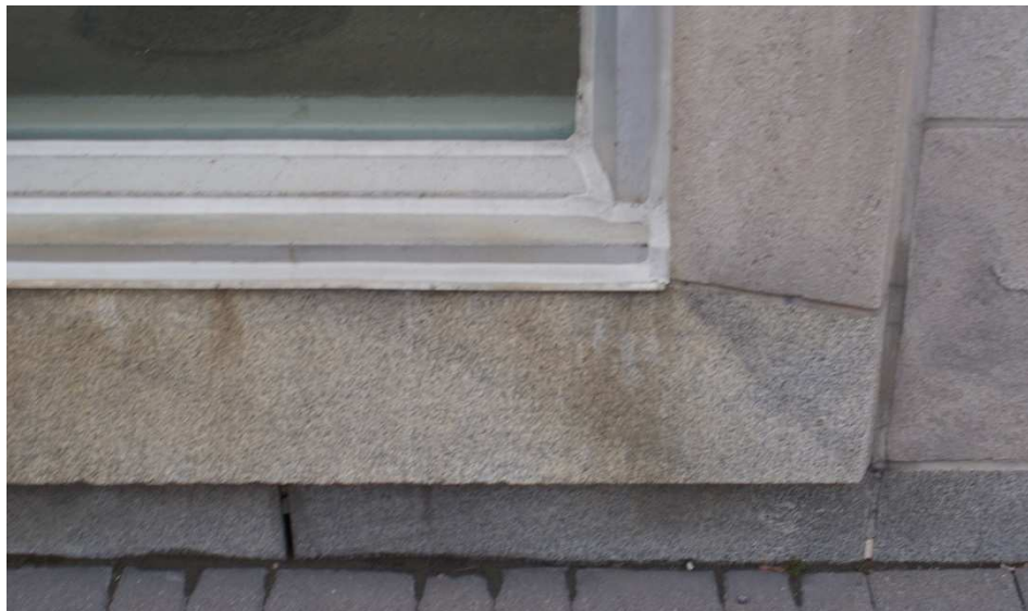
Figure 25: Detail of the granite plinth course and granite windowsill surround at the base of the three-storey Kent Street window. The colour of the granite sill is very close to the limestone cladding and window surrounds. Source: Commonwealth 2022.
