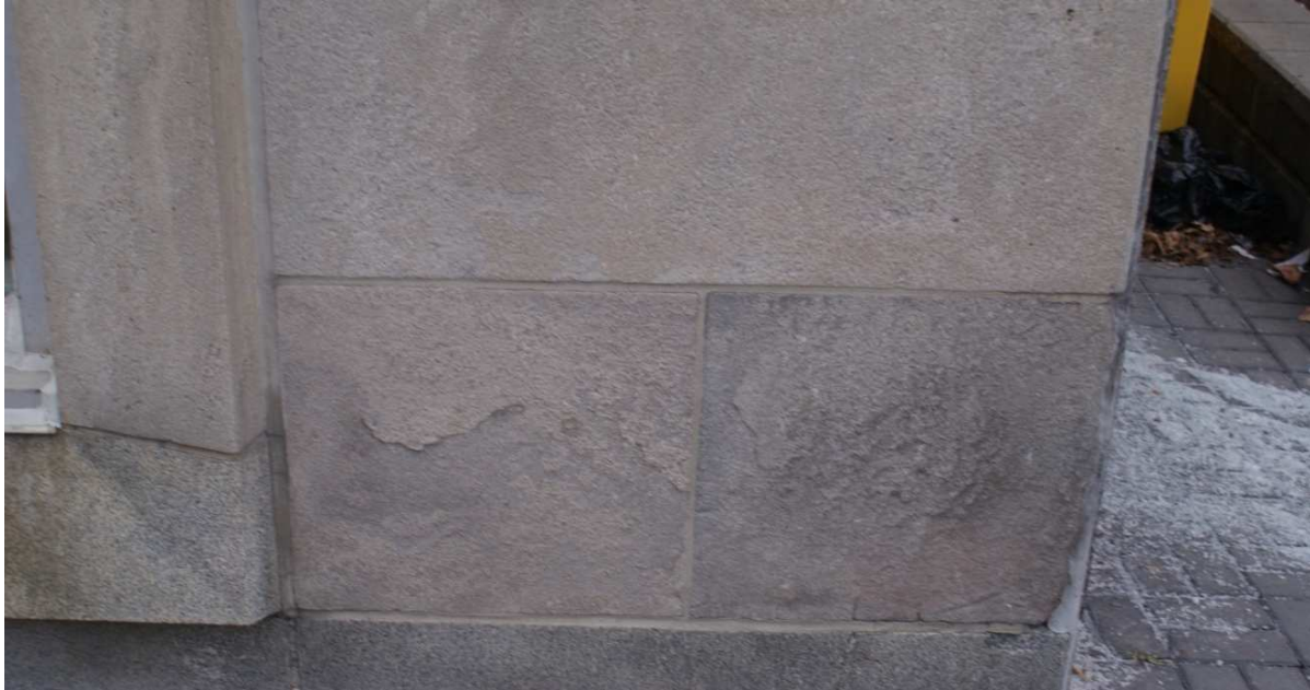
Figure 22: Detail view at the base of the wall at the south-west corner. The surface of the two Niagara limestone panels at the base of the wall are scaling due to de-icing salts. The granite plinth course is evident at the bottom of the photo. The Niagara limestone window surround is the vertical element to the left and a granite windowsill/surround below. Source: Commonwealth 2022.
