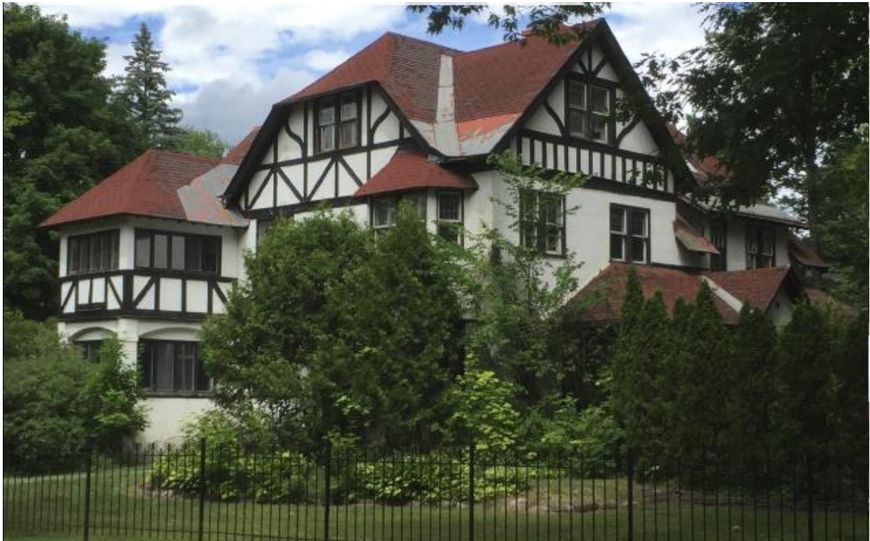
A view of the existing semi-detached from Lisgar with the two-storey sunroom/porch. Based on a comparison of the 1928 and 1965 aerial views it would appear to be an original feature. Below are views from the street documenting the bucolic landscape offering minimal visual access in keeping with picturesque principles.
