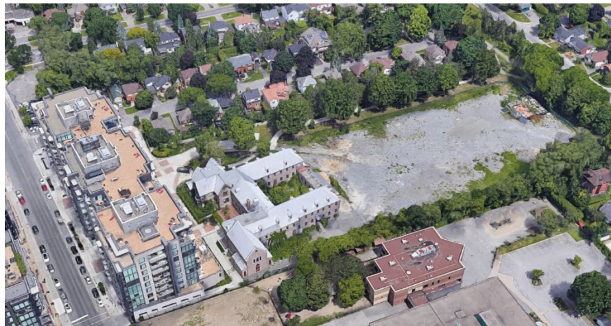
Figure 2 - View of the site post construction of Phase 1 [Google 2022].
