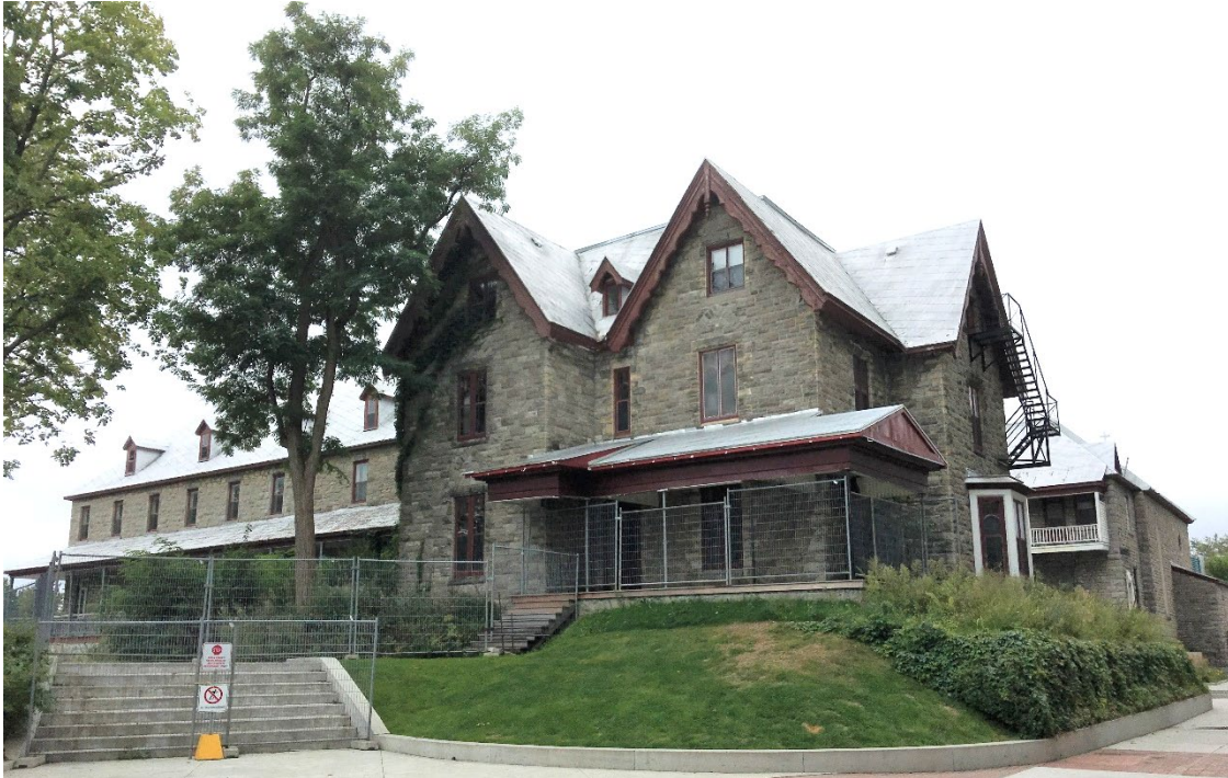
Figure 3 - The original house, north-east view (RMA 2017).
