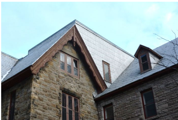
Figure 7 – Elm House/ Convent exterior connection (Photo: RMA+SH, 2022).
