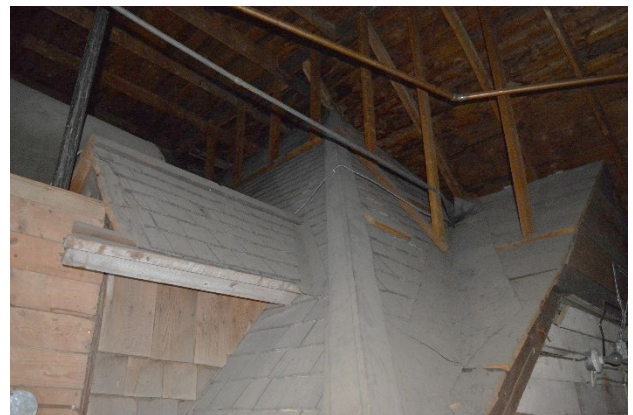
Figure 8 – Elm House/ Convent interior connection (Photo: RMA+SH, 2022).
