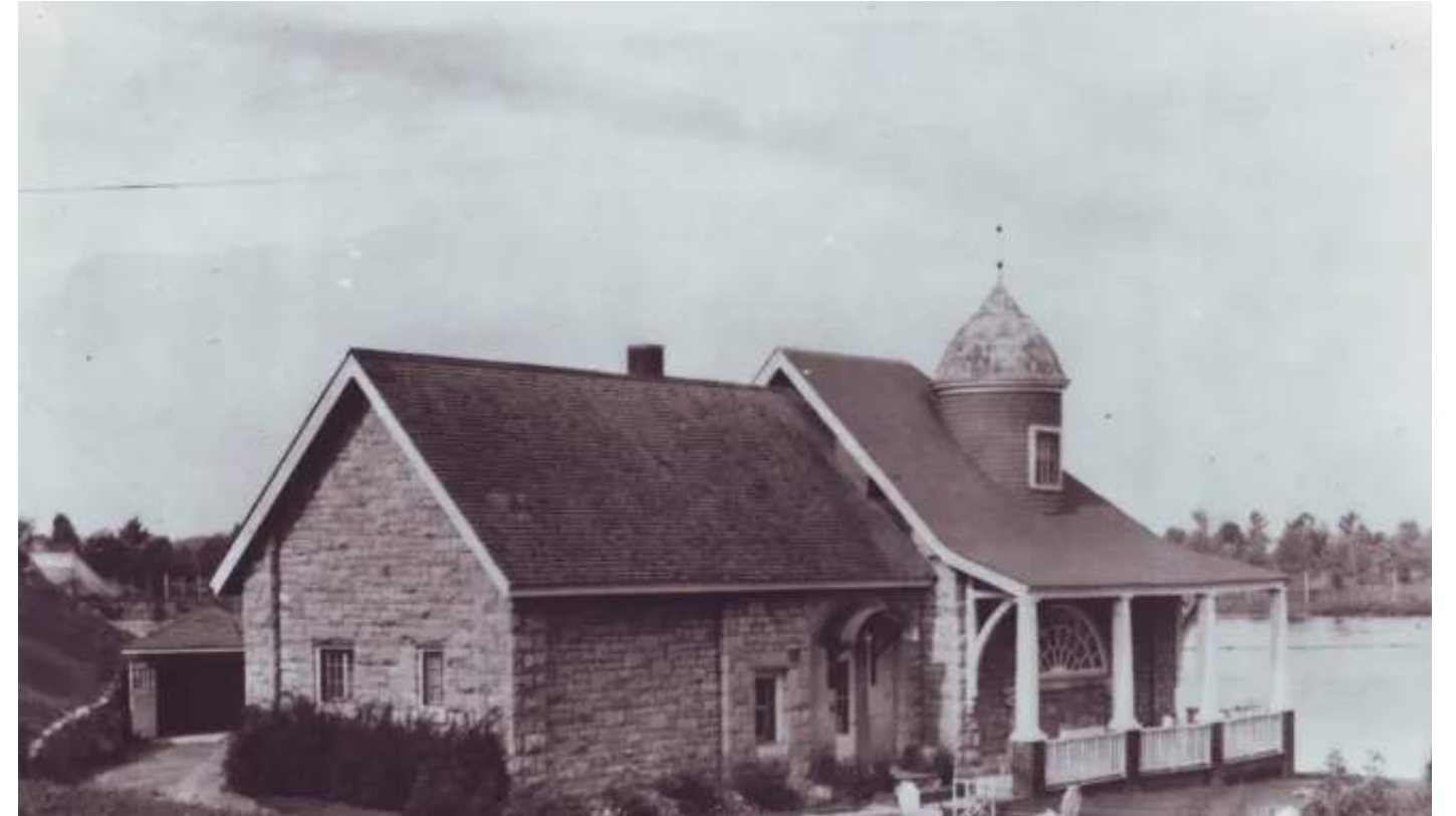
Image 1.2 View of the original building - Source: City of Ottawa
