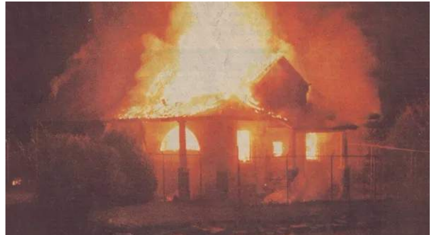
Image 1.3 Fire that destroyed the pumphouse - Source: Kitchissippi.com, 2017, originally from Ottawa Citizen
