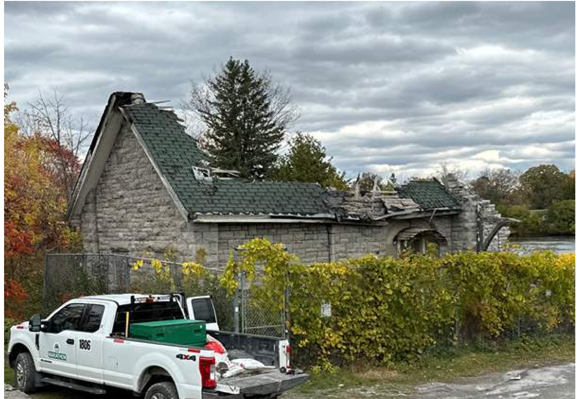
Image 1.1 View of existing pumphouse ruin - Source: CSW, 2022
