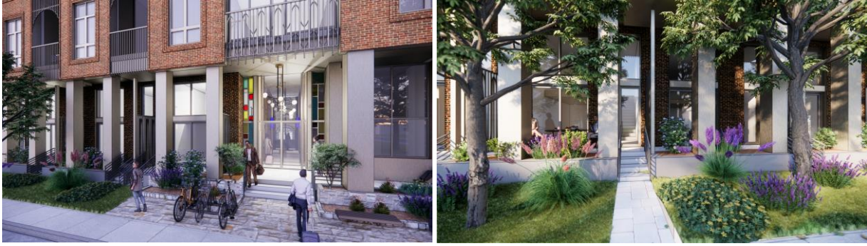
Figure 15: Detail view of the main entrance at Blackburn and ground floor entrances along Blackburn, defining the cadence along the street. Salvaged limestone from Bate Hall has been used as a facing of ground floor terraces along Blackburn. The reuse provides a link to the existing building and integrates the two facades.
