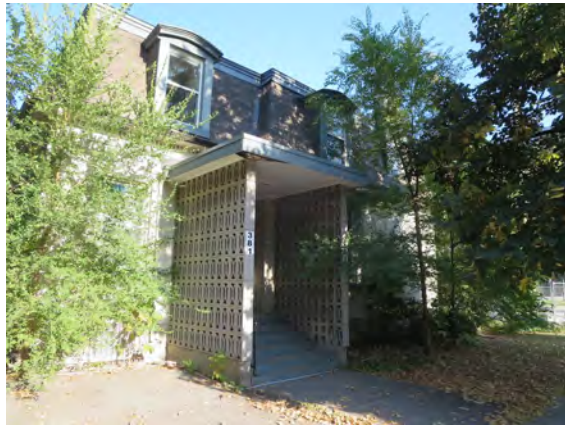
231 McLeod Street - Metcalfe Street facade with porch addition
