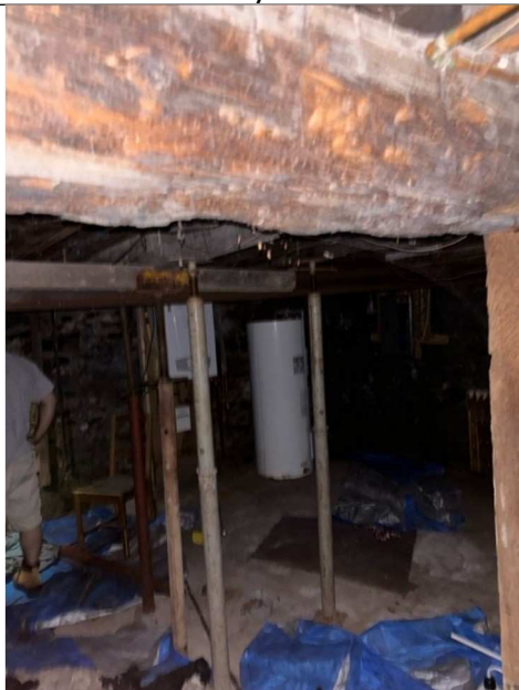
Photo 12: Temporary jackposts installed to support sagging floors.
