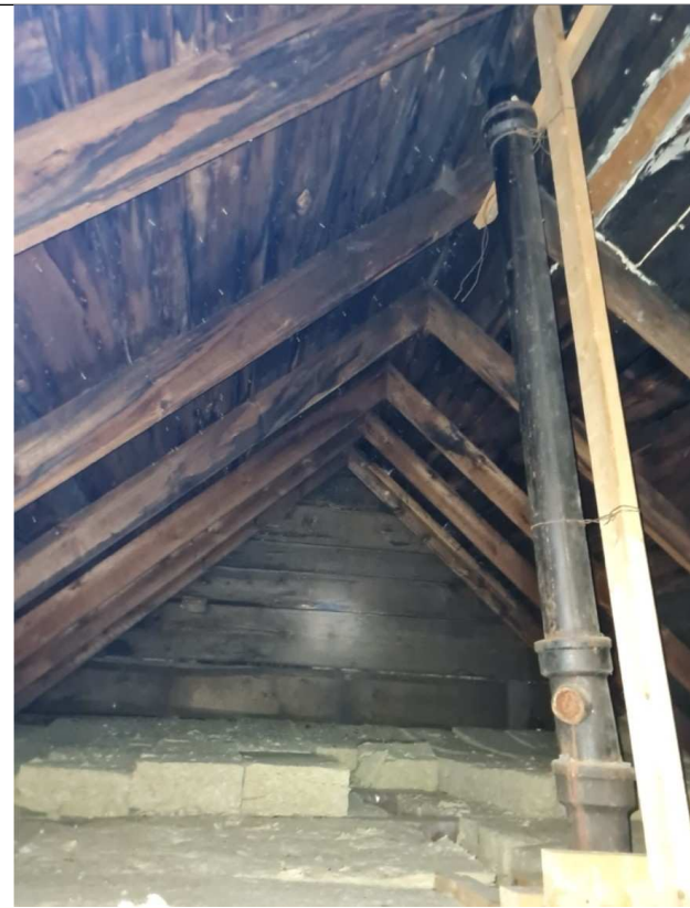
Photo 29: East gable end wall in attic.
