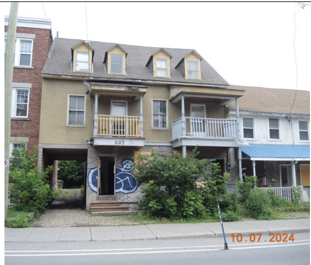
Photo 27: Roof line shows signs of sagging near the middle of the roof.
