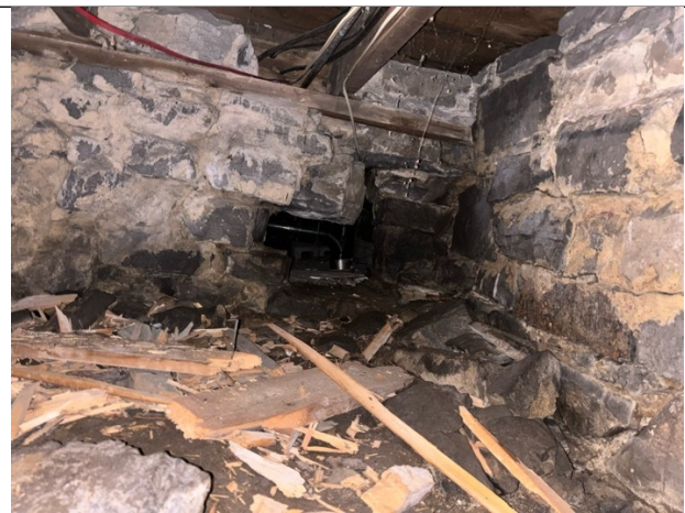
Photo 11: Opening at the corner of the foundation wall.
