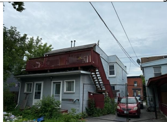
Photo 14: View of east wall and rear addition.
