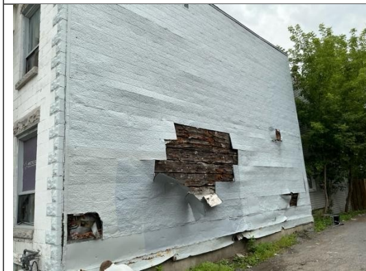
Photo 13: View of East wall.
