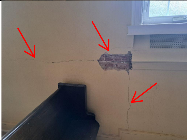
Photo 29 Cracks are noted along the left side (South) wall
