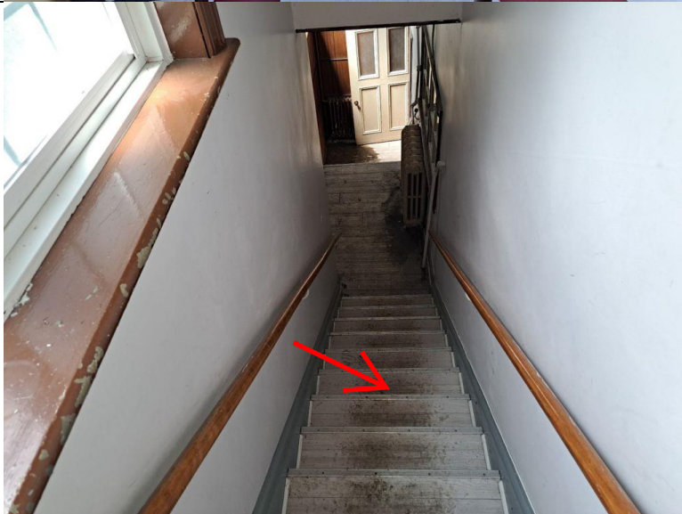
Photo 47 Staircase to the basement, covered with laminated wood
