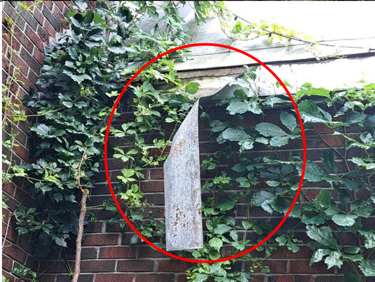
Photo 68 Flashing damage is noted
