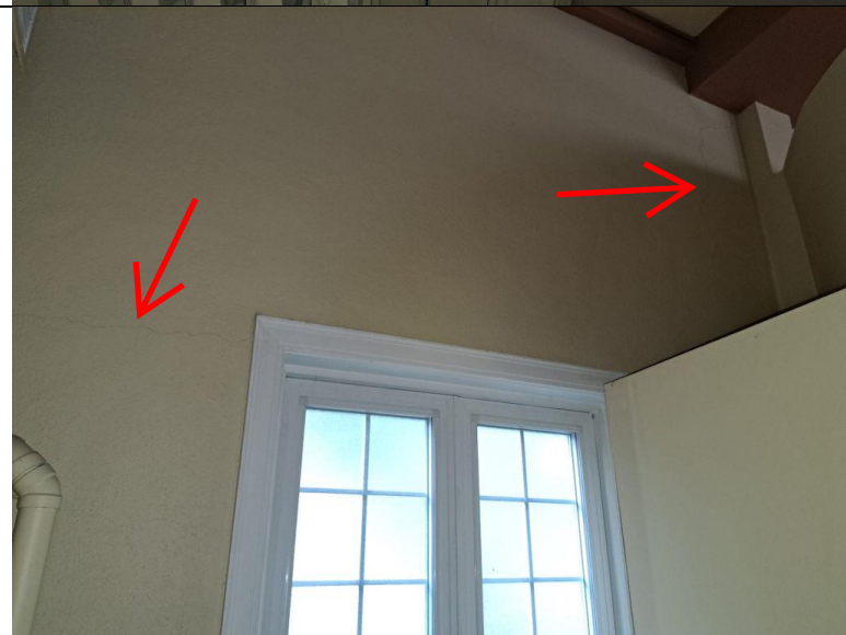
Photo 36 Several hair cracks at the top and the bottom of the windows and door lintel, and painted plaster with average quality
