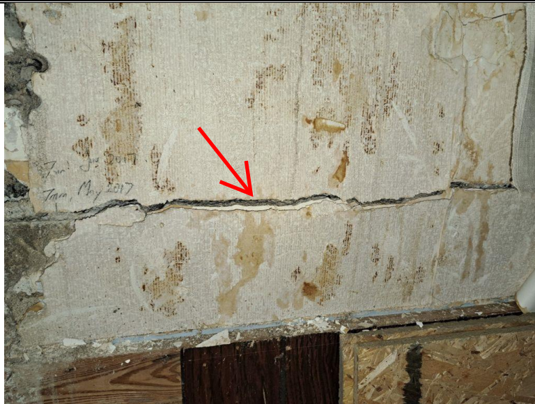
Photo 58 Horizontal crack of at least 5mm width at the rear side wall (East side) at the basement level
