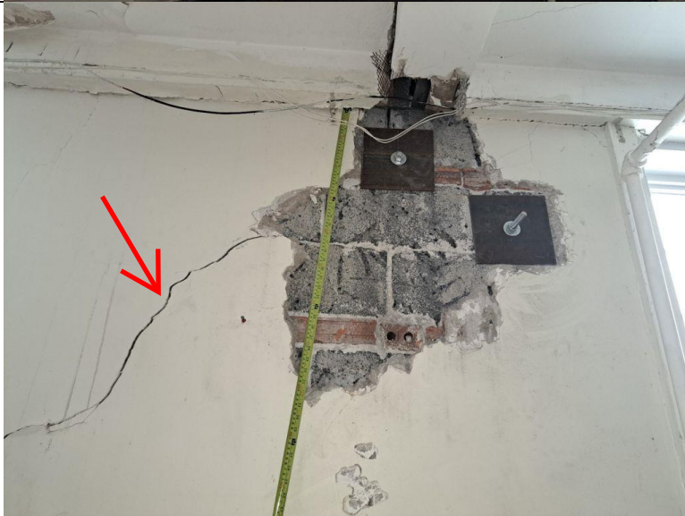
Photo 50 Diagonal cracks of 4mm width
