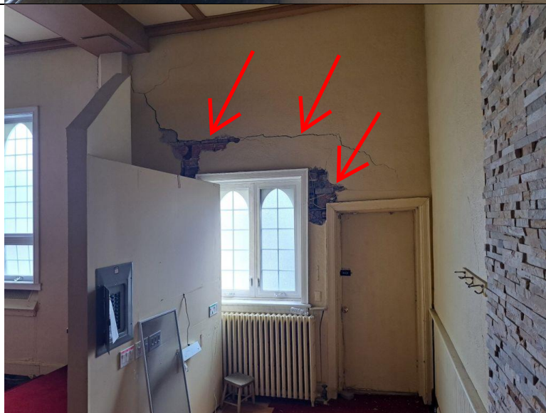
Photo 30 Cracks are noted along the left side (South) wall
