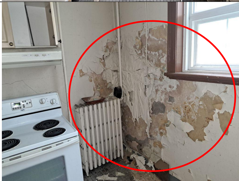
Photo 66 Moisture intrusion, paint peeling off, and water leakage on the floor
