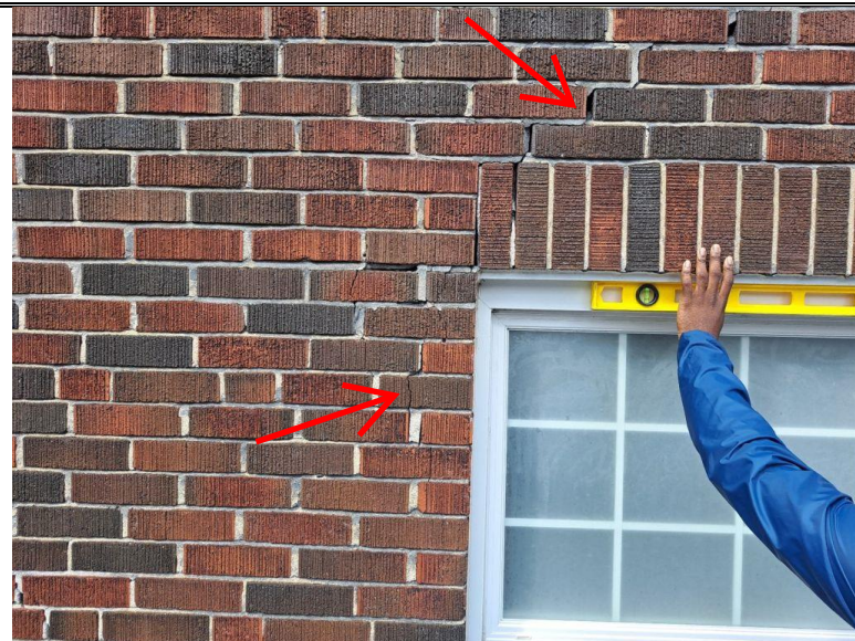
Photo 10 Stepped wide cracks noted along the South wall
