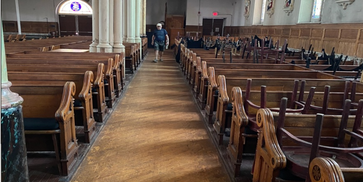
Figure 9. West Aisle showing pews anchored to raised hardwood flooring
