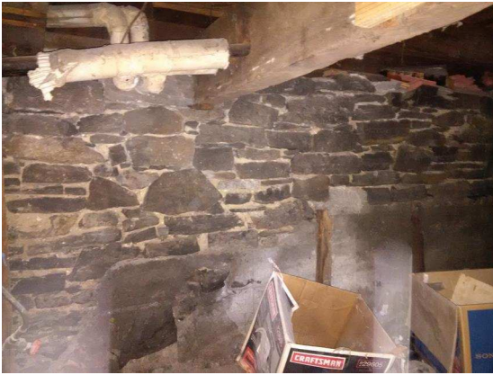
Photo Four – Rubble Stone Wall
