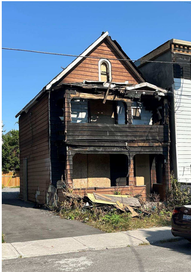
79 Guigues – South Elevation Viewed From Guigues Street
