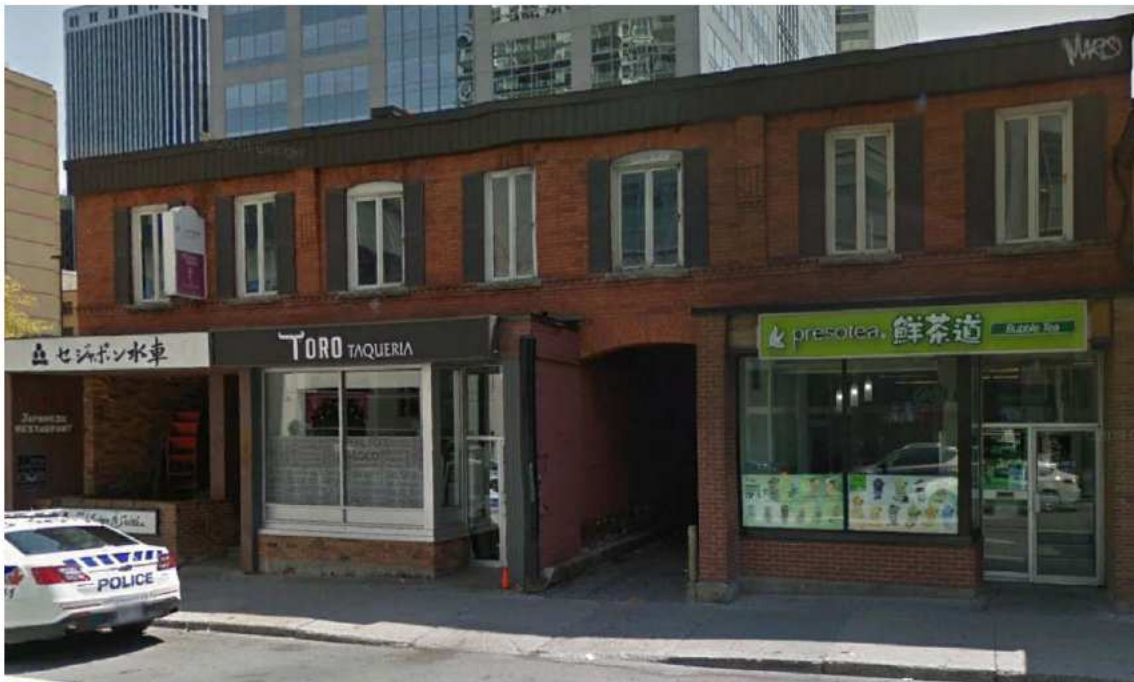
Figure 4: View of the 3-bay façade articulated with projecting pilasters that group the bays into a 2:3:2 fenestration pattern. The central bay is further articulated with a central flat headed window flanked by two wider windows with segmental brick arches and accented with raised pilasters and a corbelled brick band below the second floor window. The loss of the third floor and the ad hoc additions on the ground floor have lessened appreciation of this early well designed row house. Source: Google Earth.
