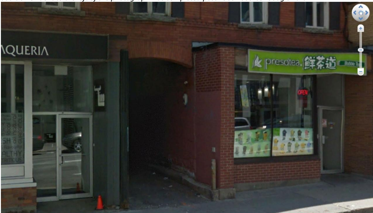
Figure 8: Detail view of the storefront on 208-212 Slater. It would appear that the projecting brick walls, and panel below the storefront window, are contemporaneous with a more recent rehabilitation of the storefronts
